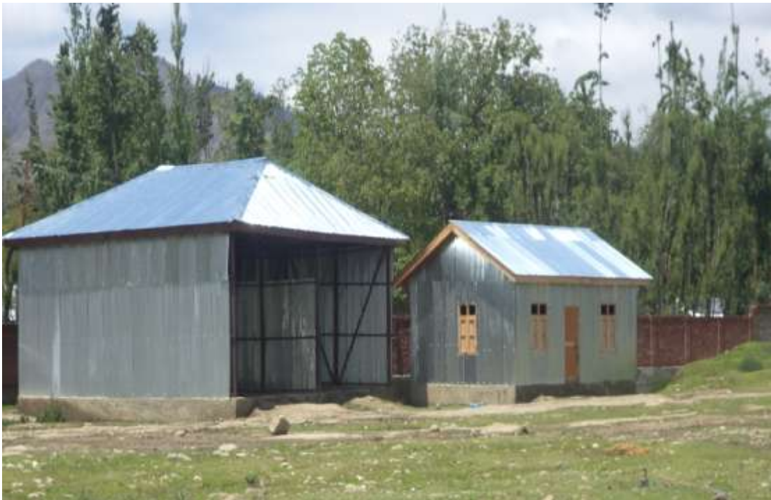
Tin sheds erected on the left side of the proposed entrance of main gate of the College
