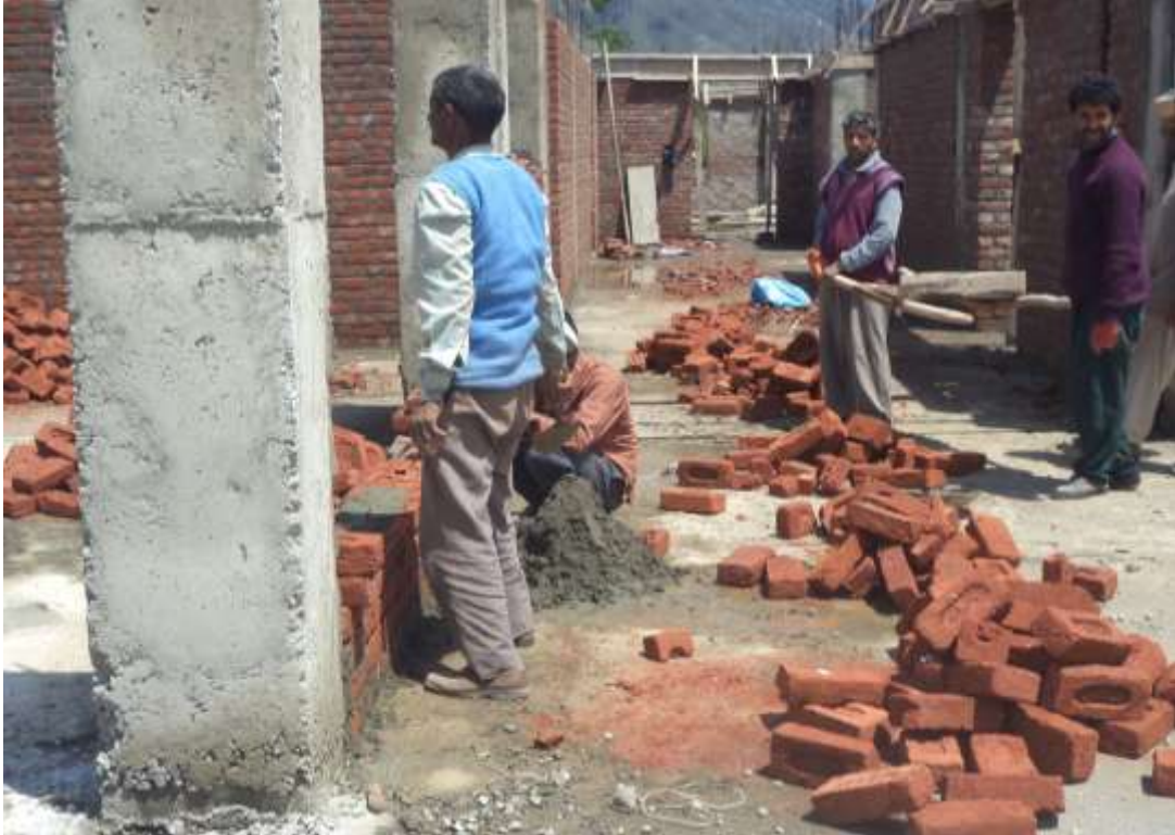
(Left wing)- Brickwork of first floor in progress
