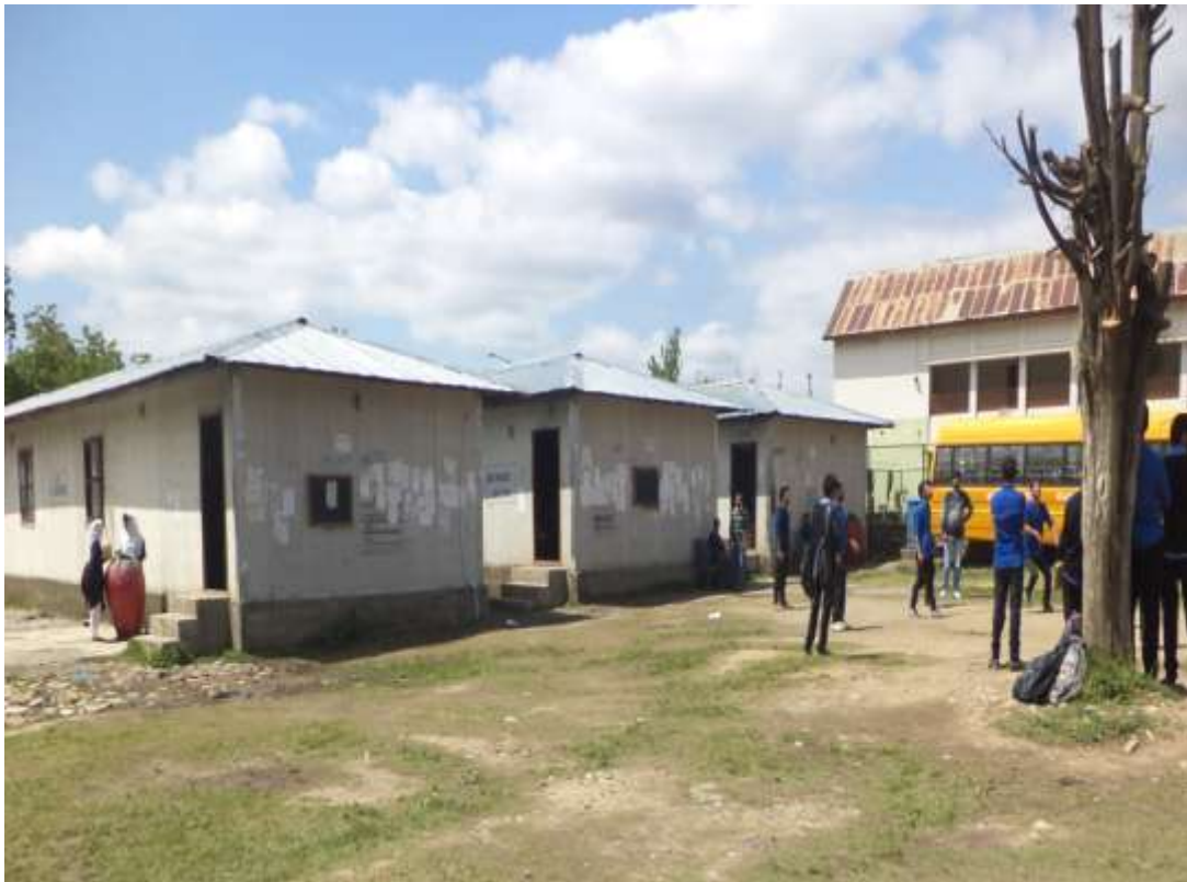
Prefab huts erected within the HSS premises wherefrom Degree College is presently functioning.
