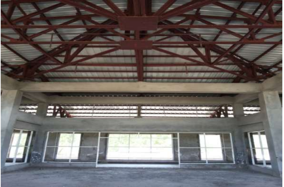
Steel Truss being laid over 1 st floor of Club Building
