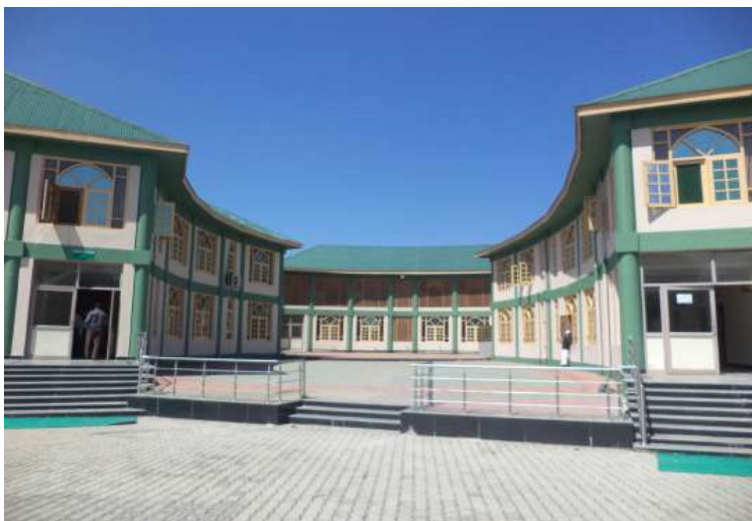
Almunium alloy door frames and stainless steel railings provided/ fixed along ramp on the entrance of CFC
