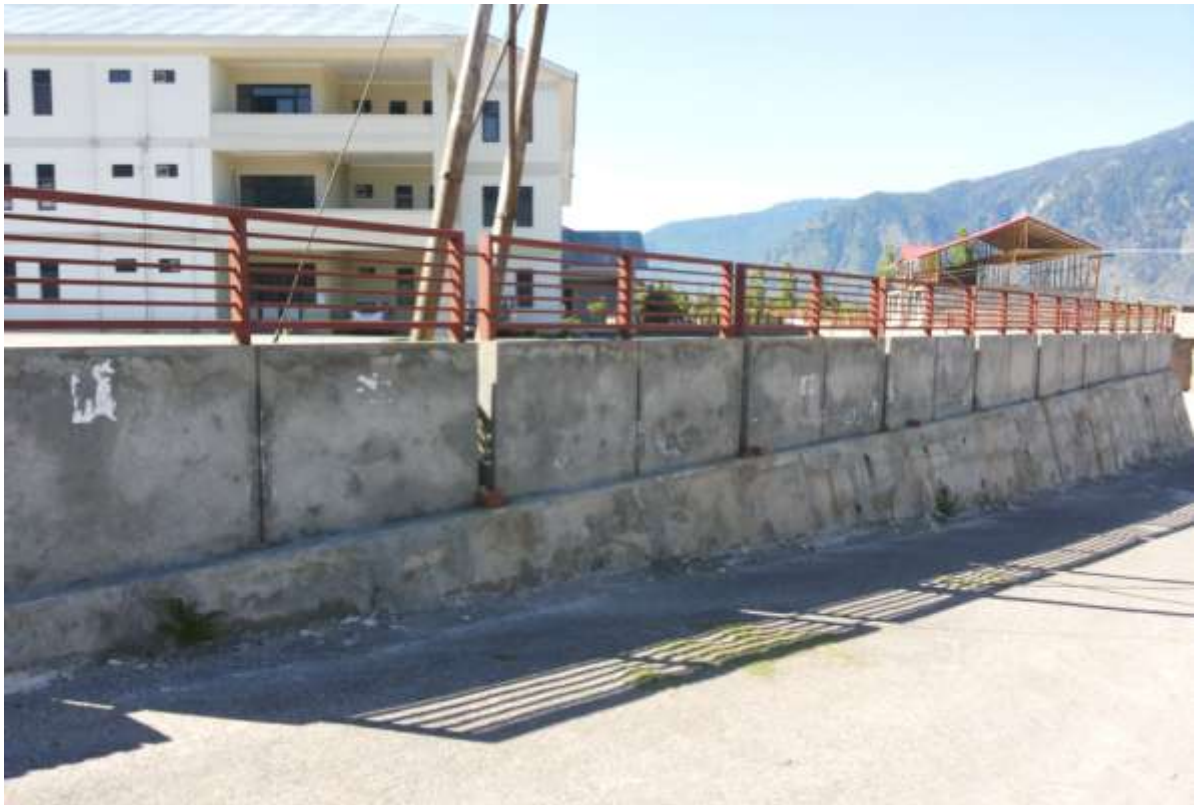
Boundary wall constructed on front side of complex
