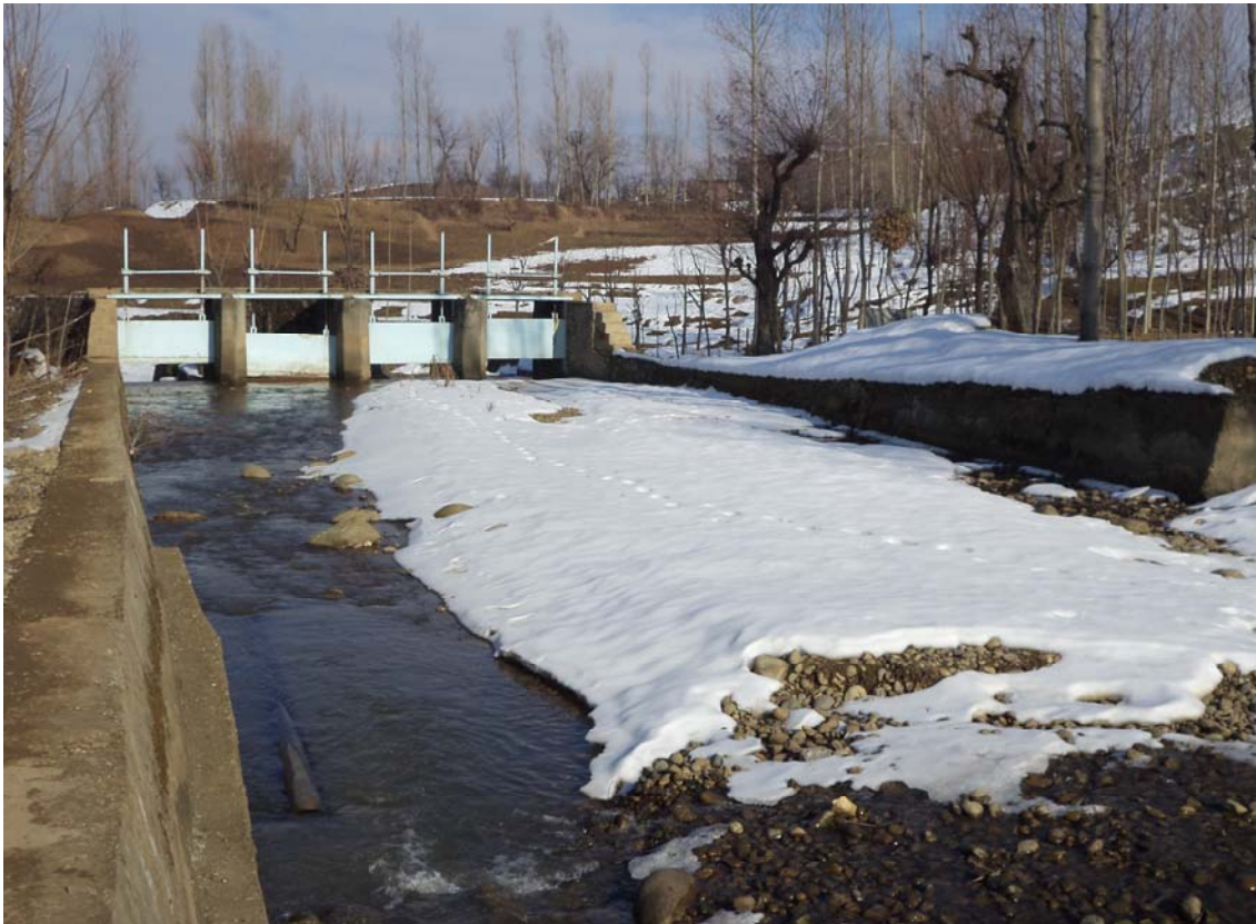
Head regulators for Kati and Karshan branches of the canal
