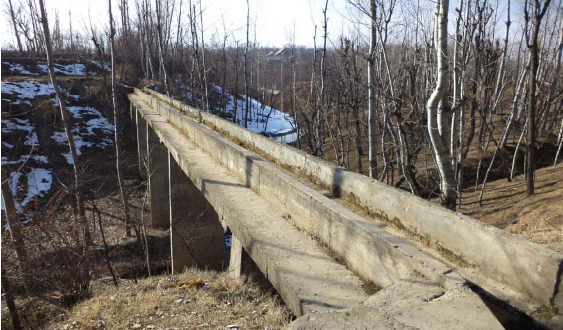
RCC flume constructed on one of the distribution network channel
