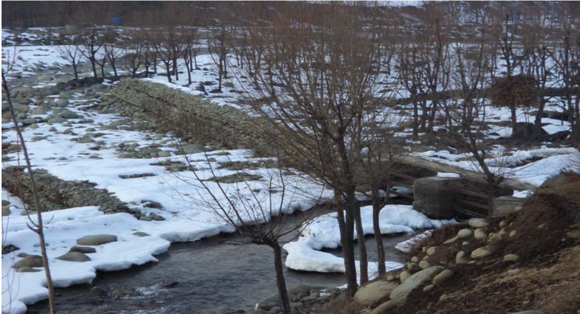
Crate work provided on the canal for protection
