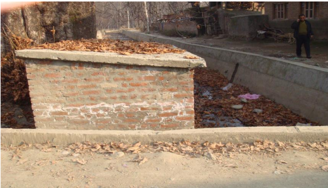
Bathroom/toilet constructed by RDD in the middle of canal at village KAHIGAM
