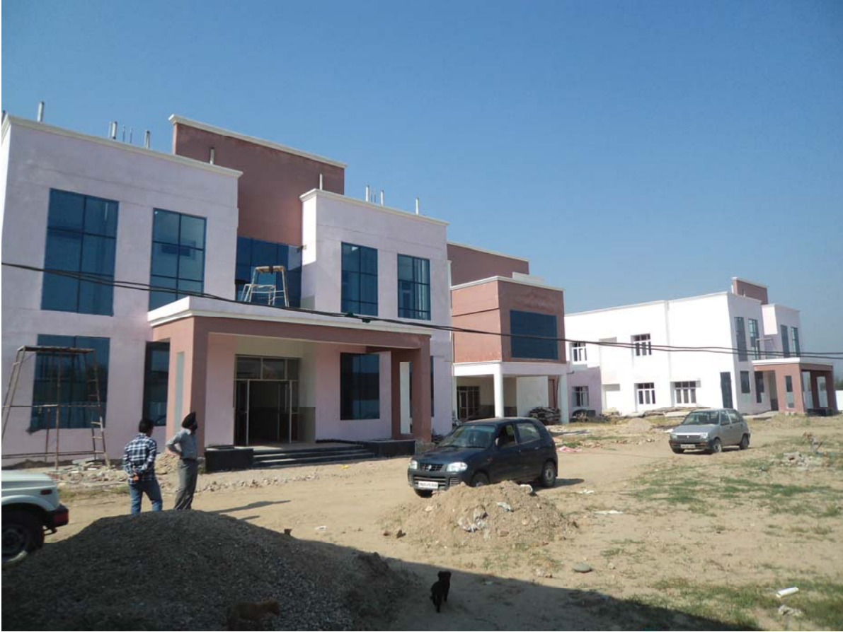
Front view of the hospital building
