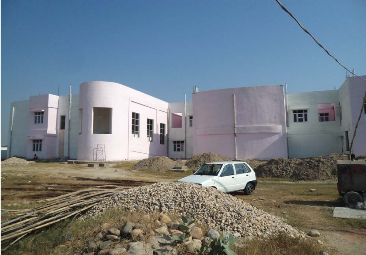
Rear view of the hospital building
