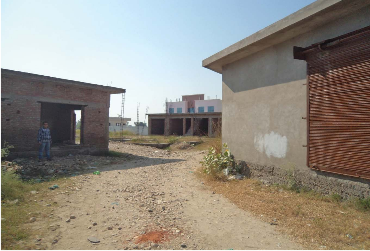
Sharp bend on the approach road
