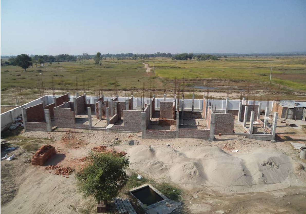
Construction work of staff quarters in progress
