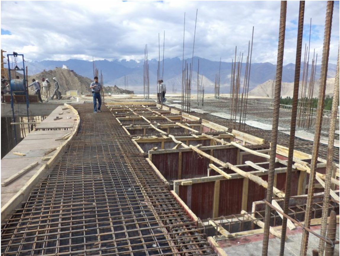
Laying of Slab for ground floor under progress
