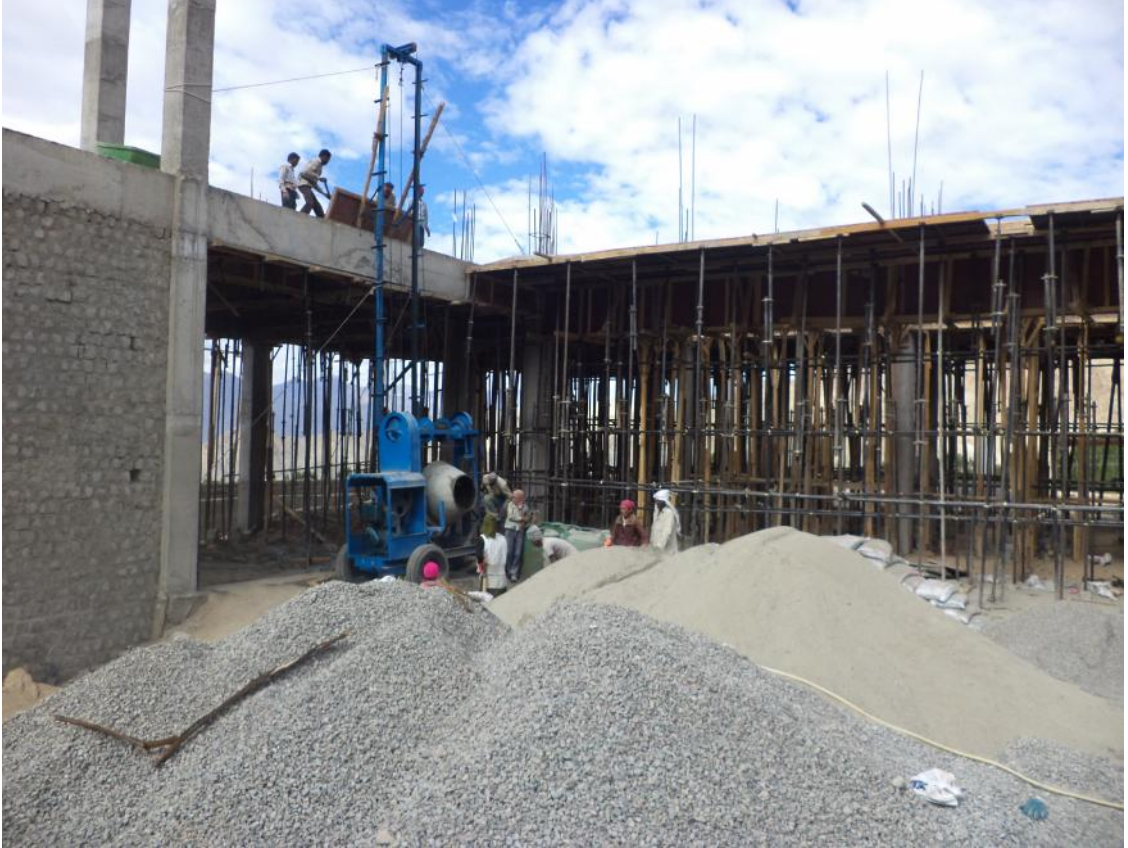
Men & machinery at work
