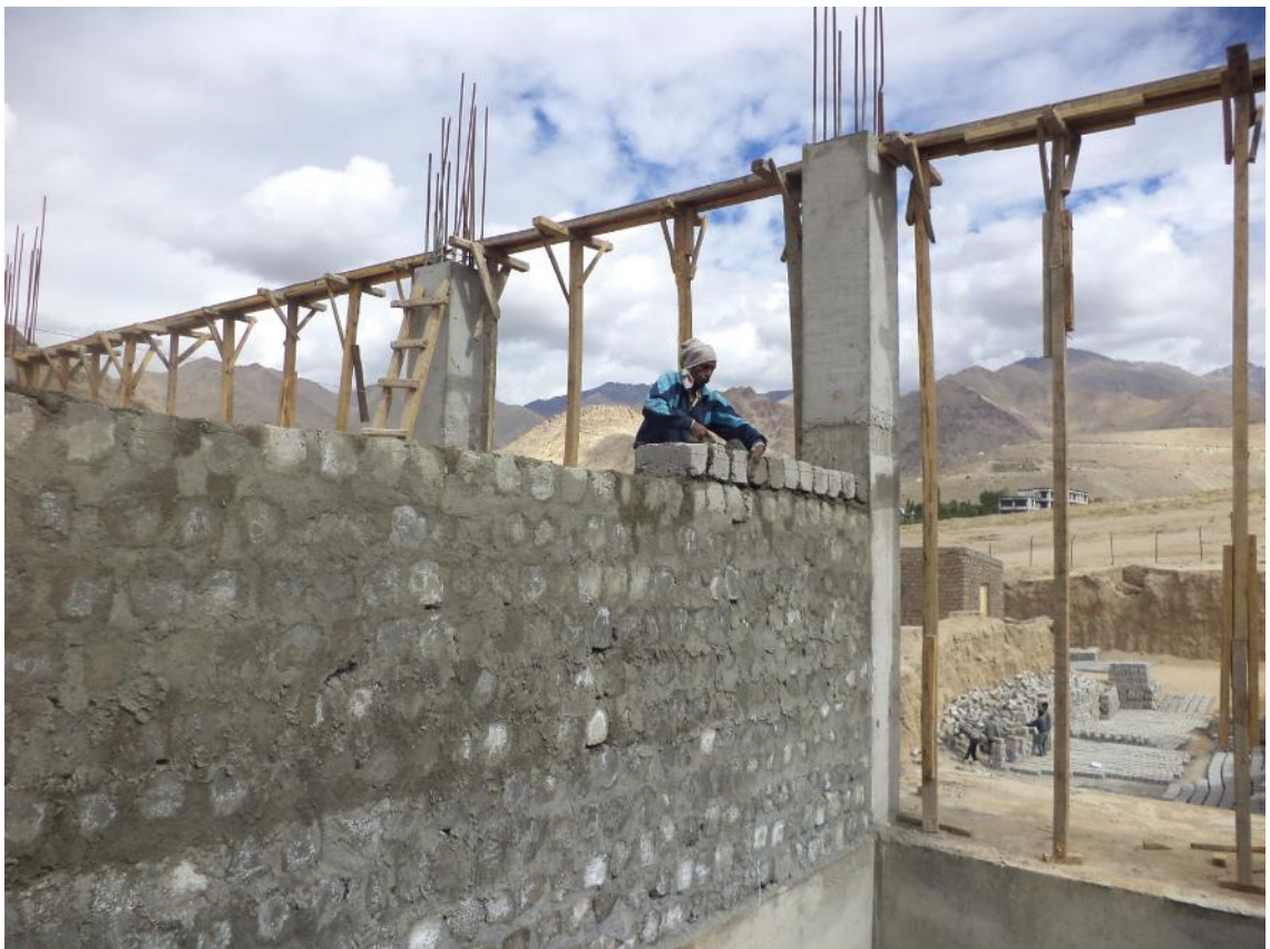
Brick work under progress
