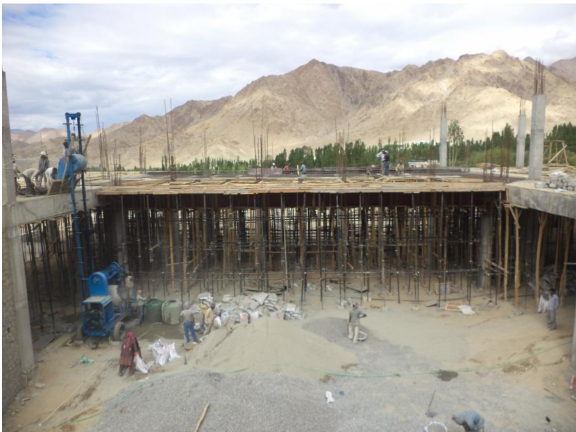
Laying of Slab for ground floor under progress
