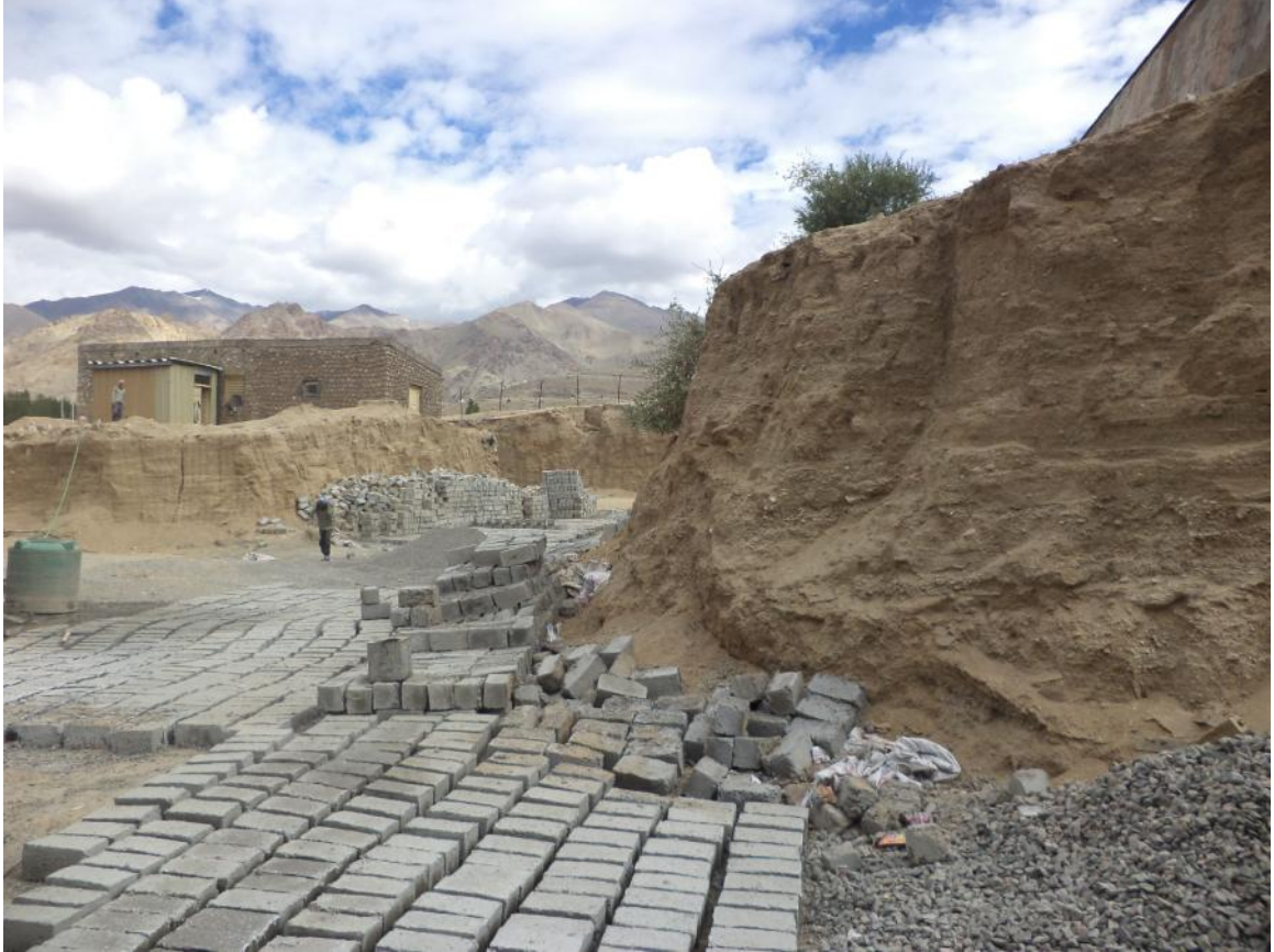
Earth cutting work done near hill toe
