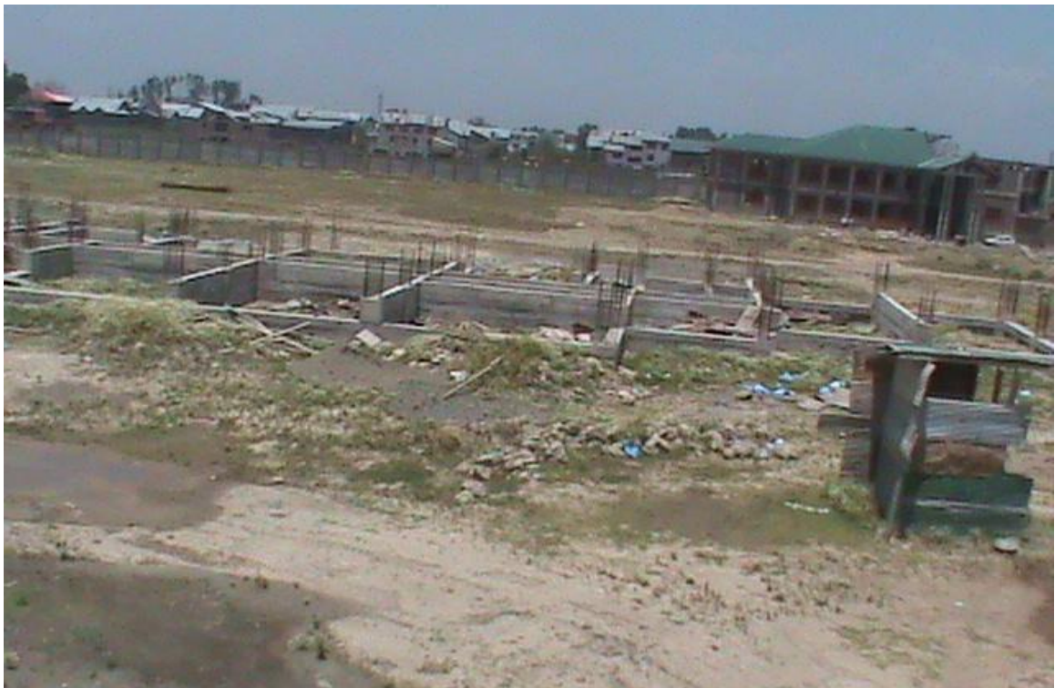
Foundation laid in Additional Services Block
