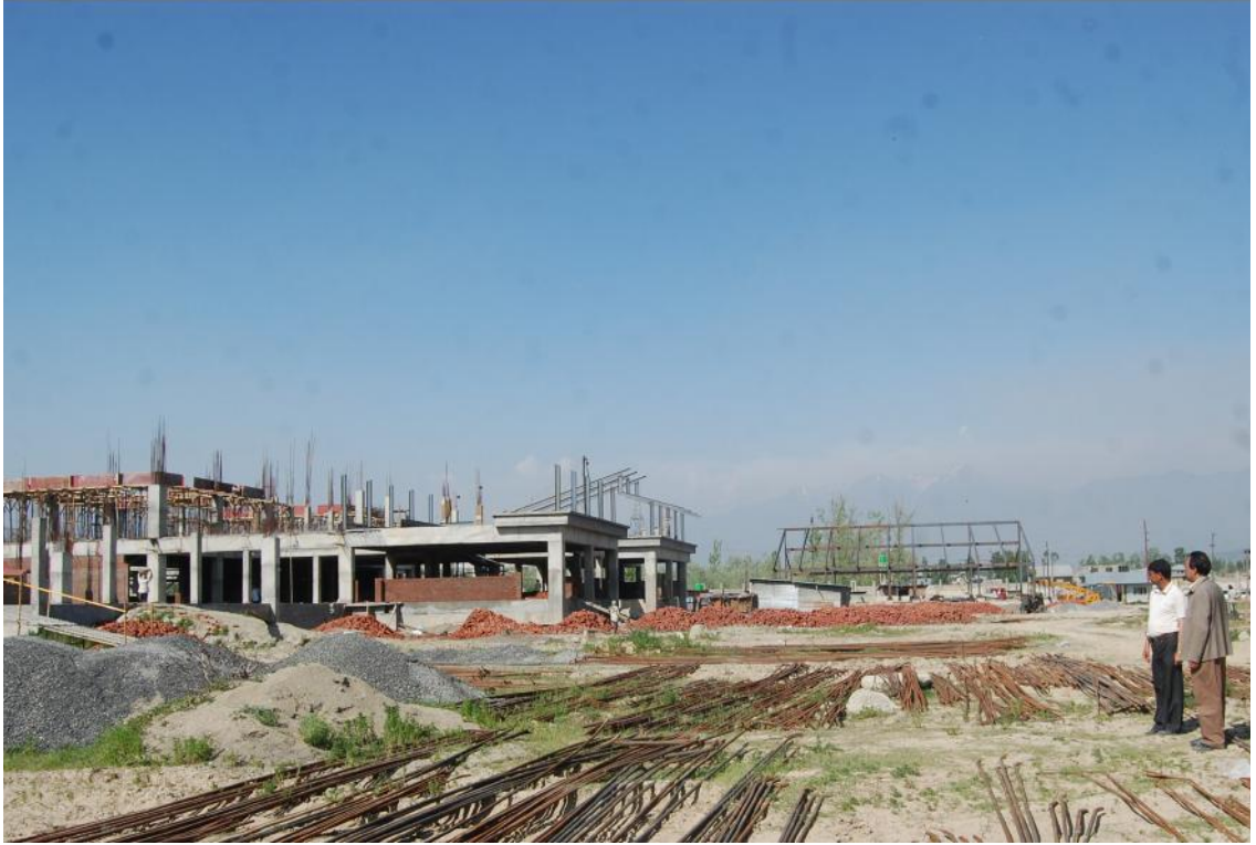
View of the N1 block, under construction
