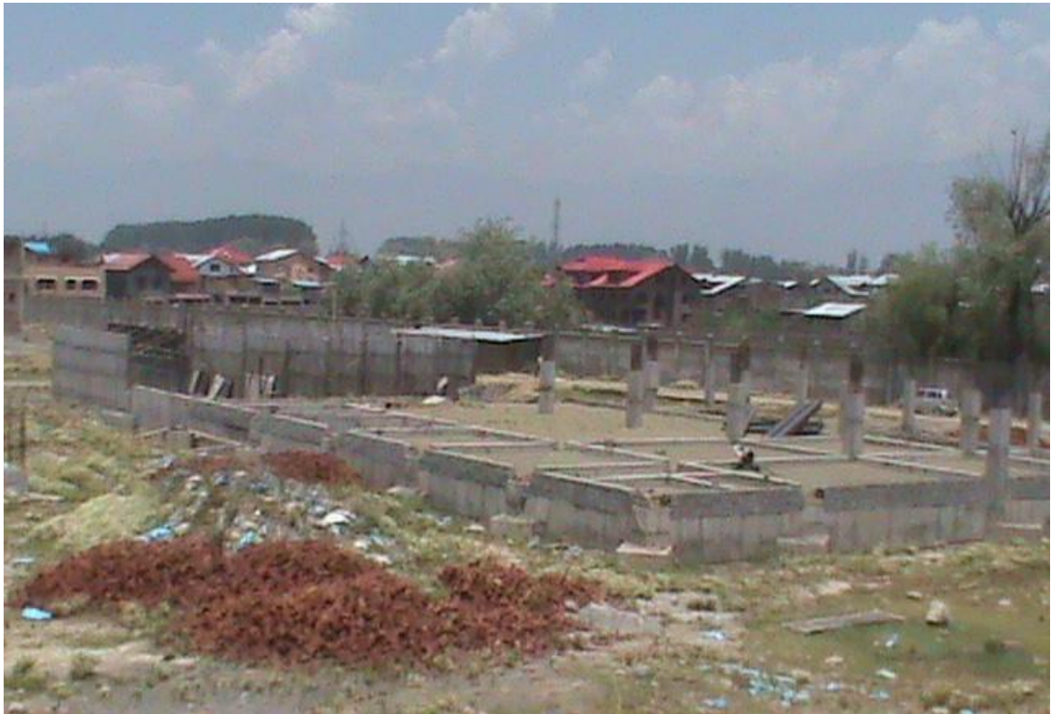
Foundation laid in Services Block
