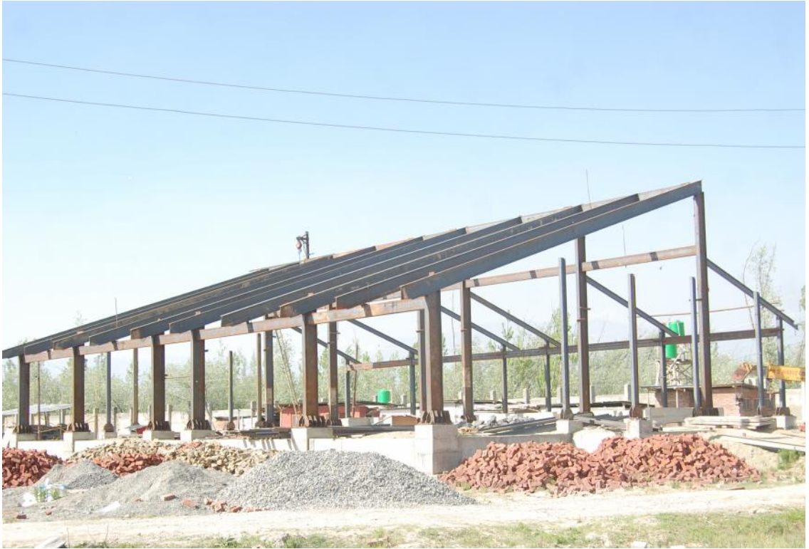
Under construction Food Court
