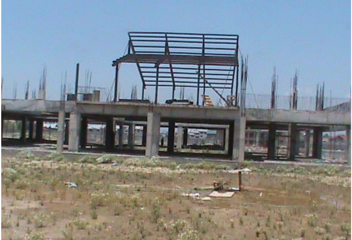
Front view of the N 3 block
