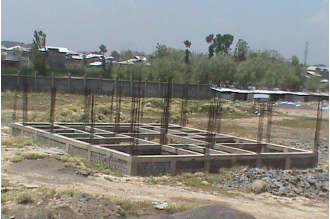
Foundation laid in judicial lockup Block
