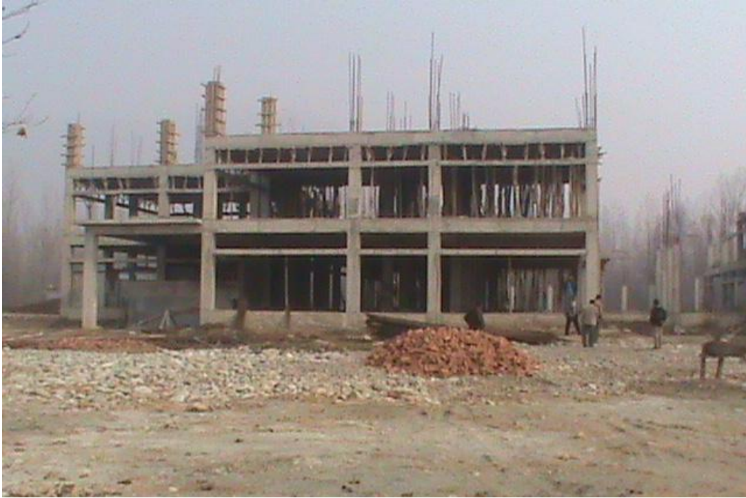
Block A – Slab over 1 st floor in progress
