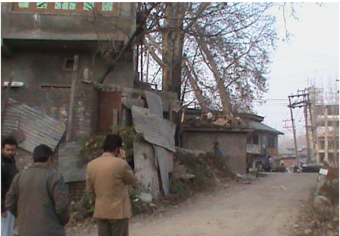
Structures near culvert, Dudrhama, coming in the alignment of the approach road at off-take point
