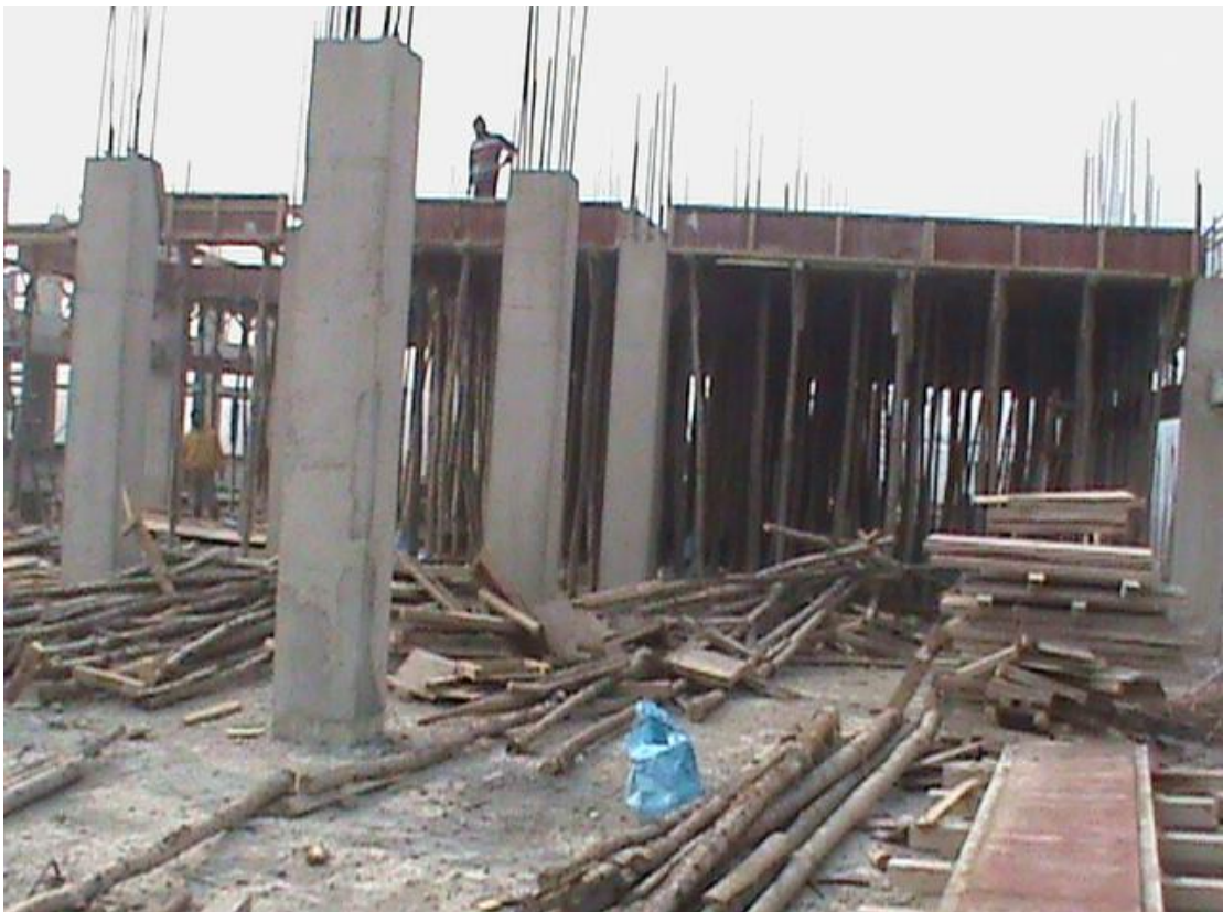
Shuttering for 1 st floor of the Block-A underway
