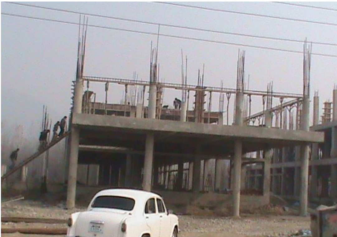
Block B – Slab over 1 st floor in progress
