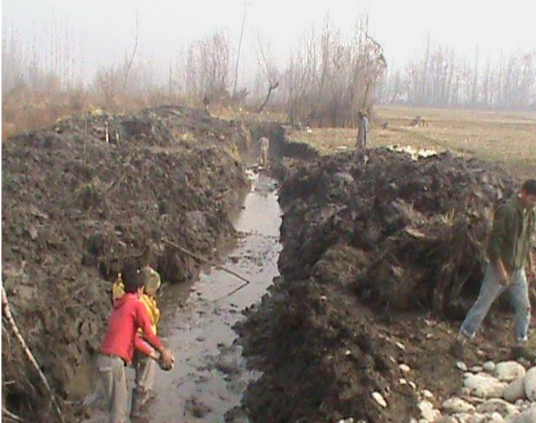
Laying of boulders in the open trench of boundary wall
