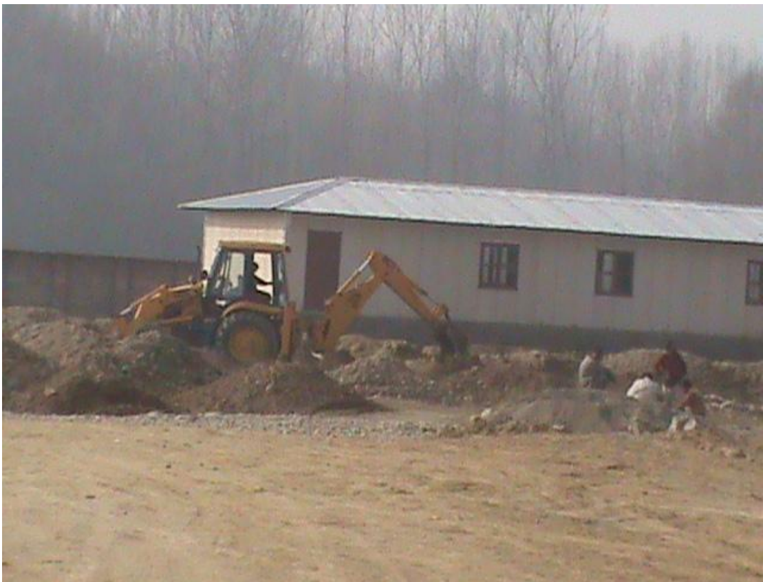
Land development work in progress
