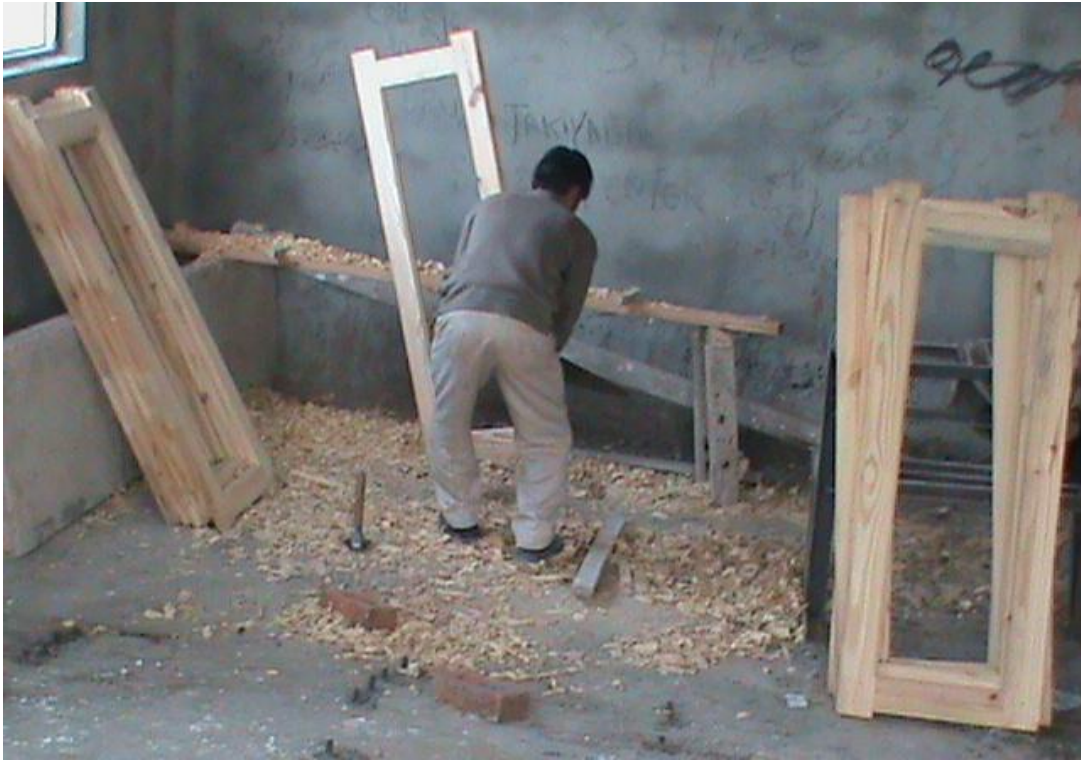
Fitting and fixing of window shutters in progress
