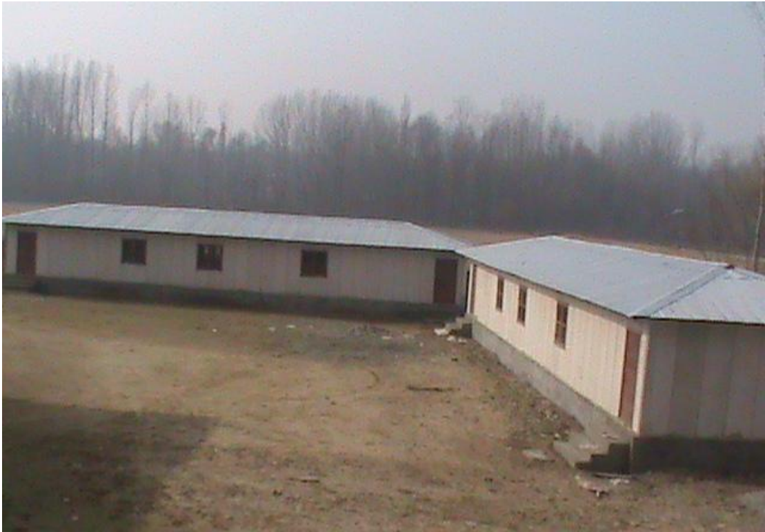
Prefab huts constructed within the college premises
