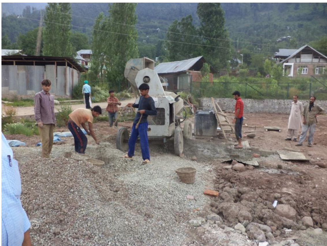
Site development works under progress
