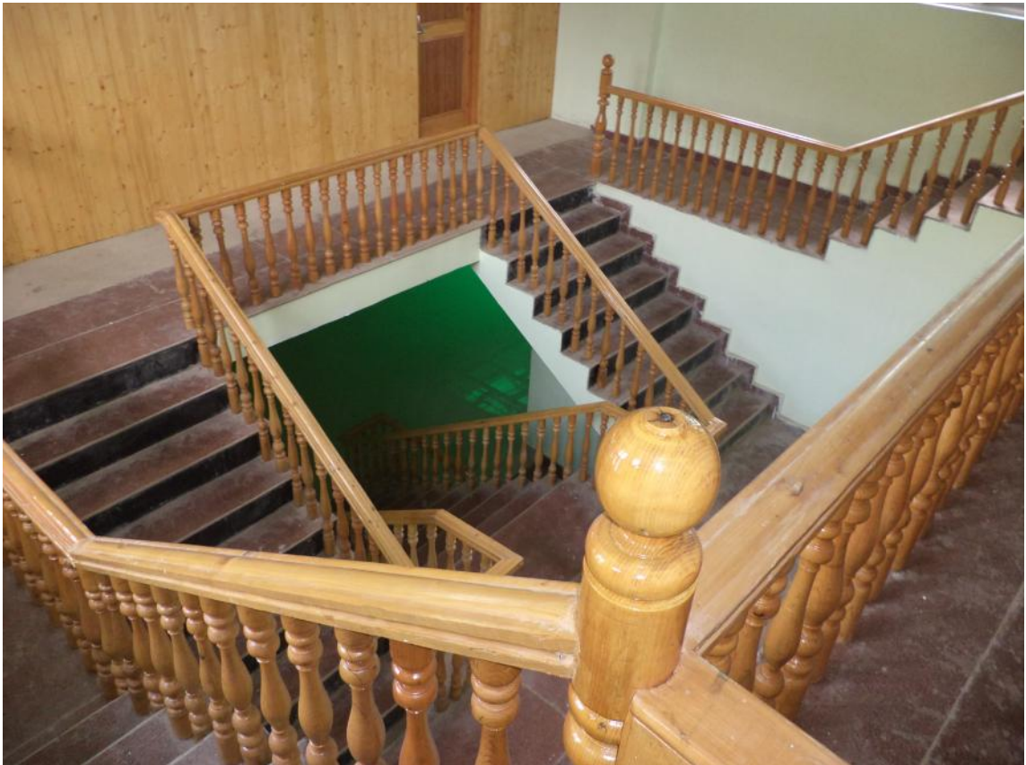
View of the stair with wooden railing
