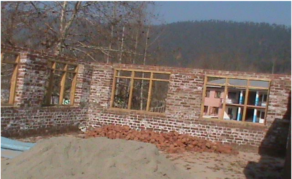
Brick work of 1 st floor completed upto lintel level
