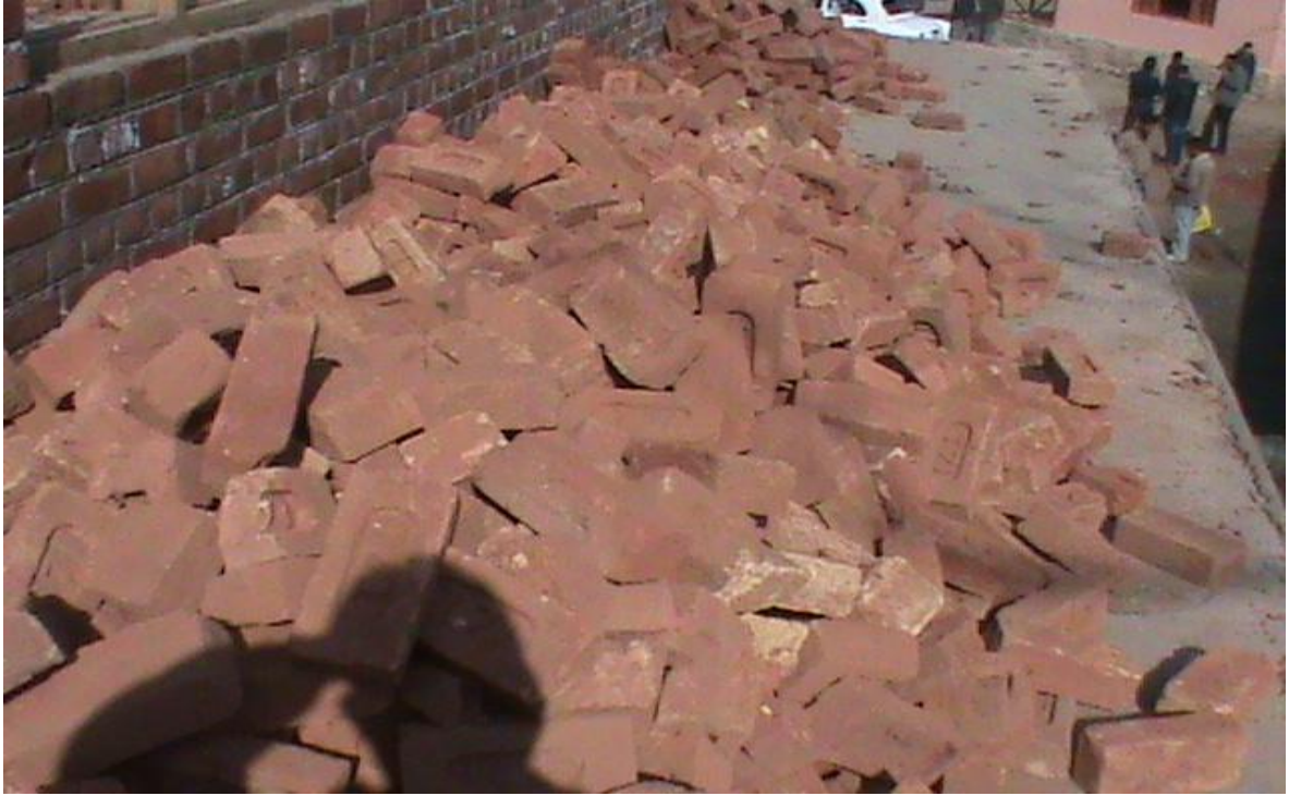
Bricks dumped on the site of the construction
