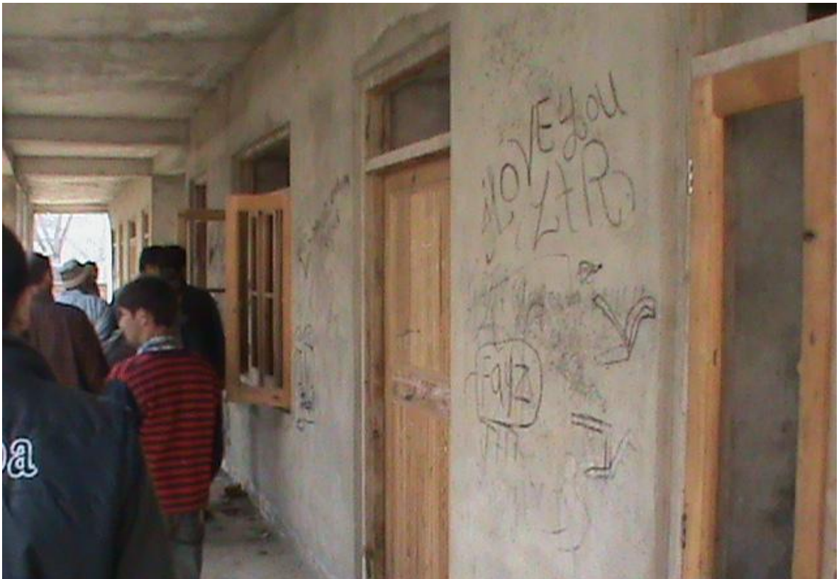
Windows/door shutters made of deodar fixed in the ground floor
