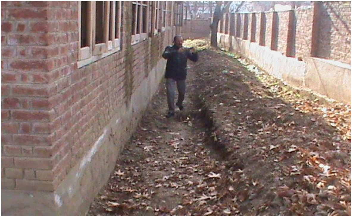
Earth excavation done to make the plinth work visible
