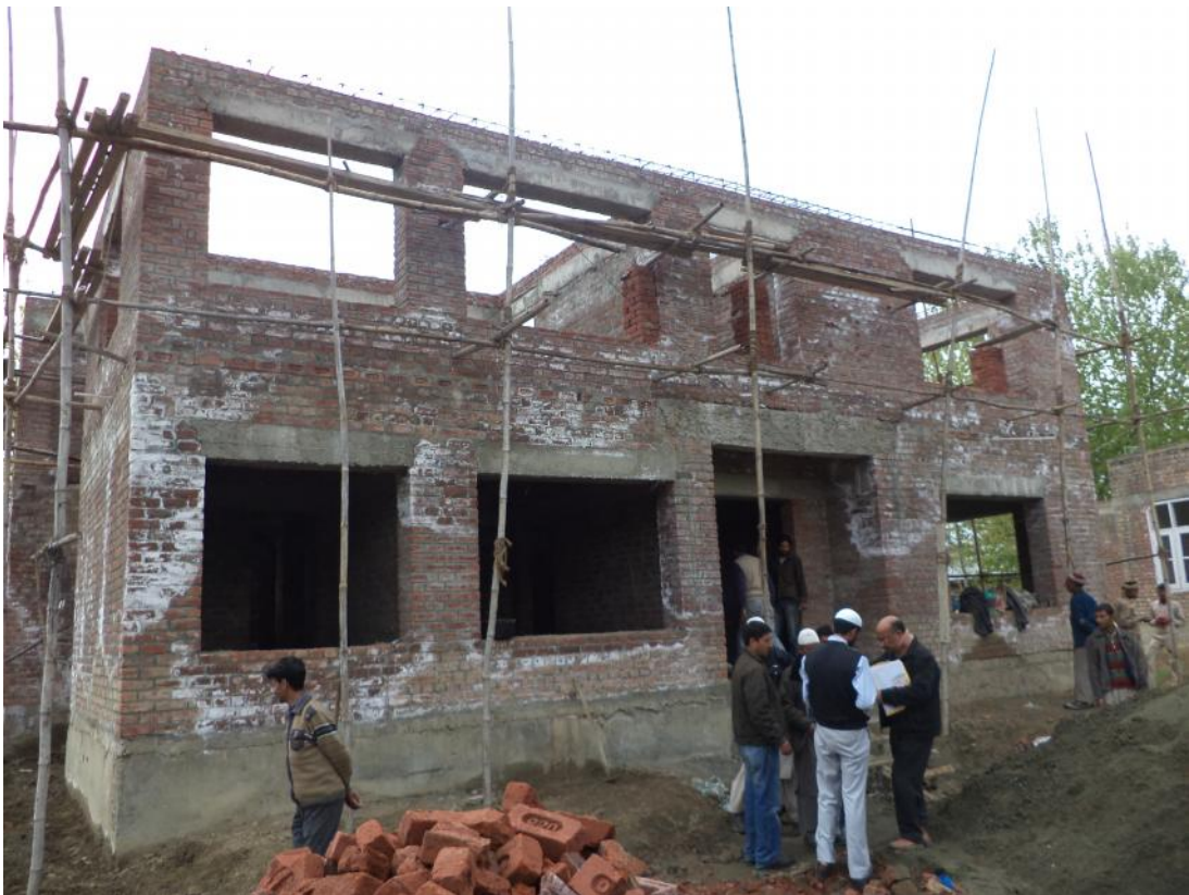
View of the Hostel Block under construction
