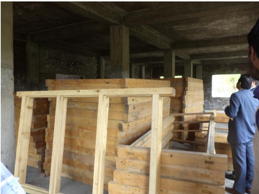
Deodar wood door/window frames for workshop building
