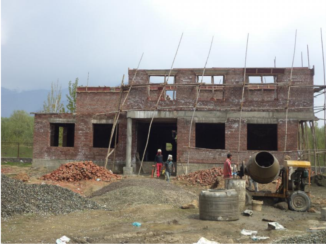
Administrative Block under Construction
