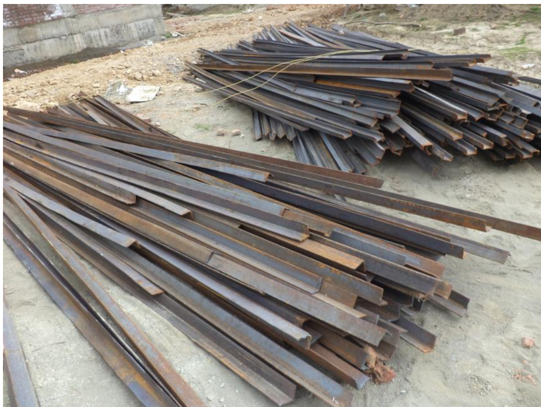
Structural steel lying at the construction site
