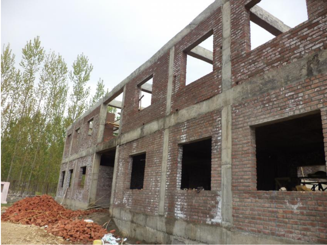
Workshop Block under construction
