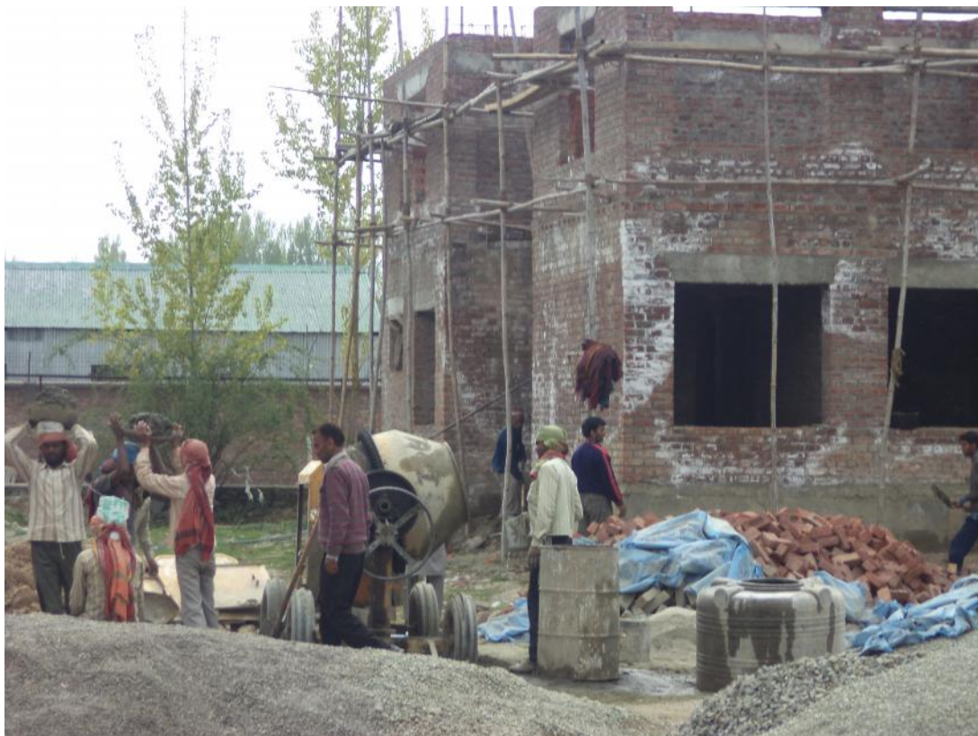
Men & Machinery at Work
