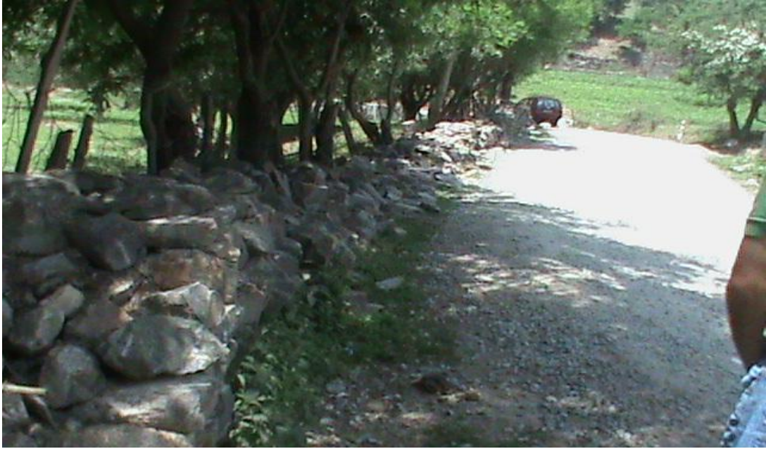
Parapet of dry stone masonry erected along side the road
