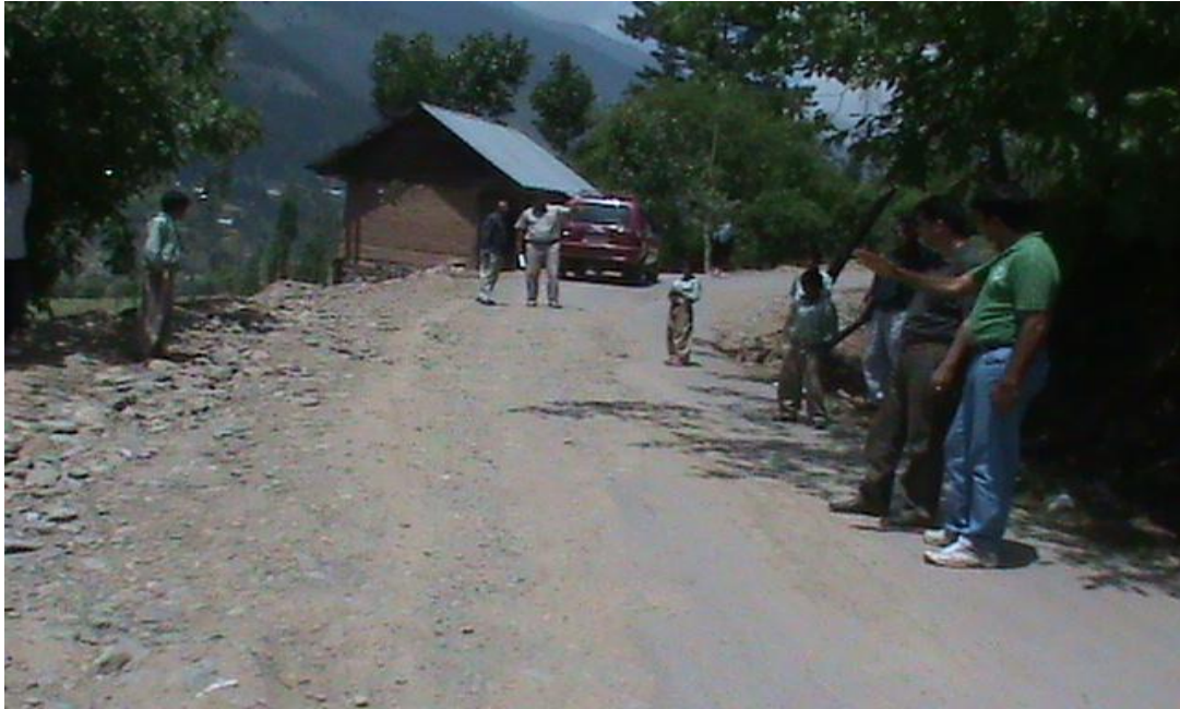
Soil/road erosion taking place due to seepage of Waniarm canal
