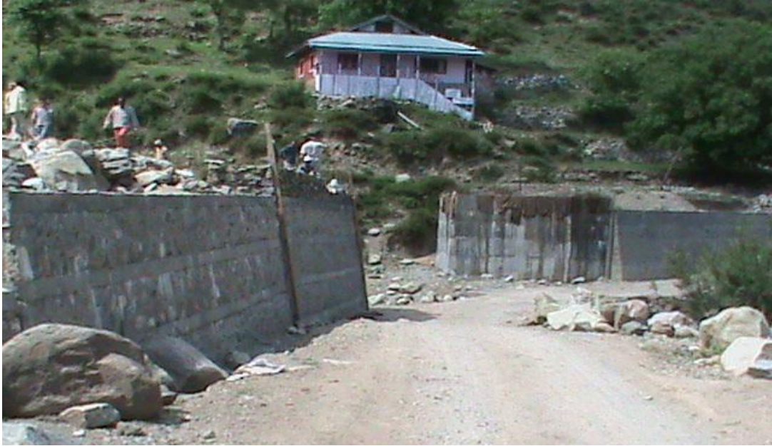
Abutments and caps laid, bridge at Km 16 at Naranag
