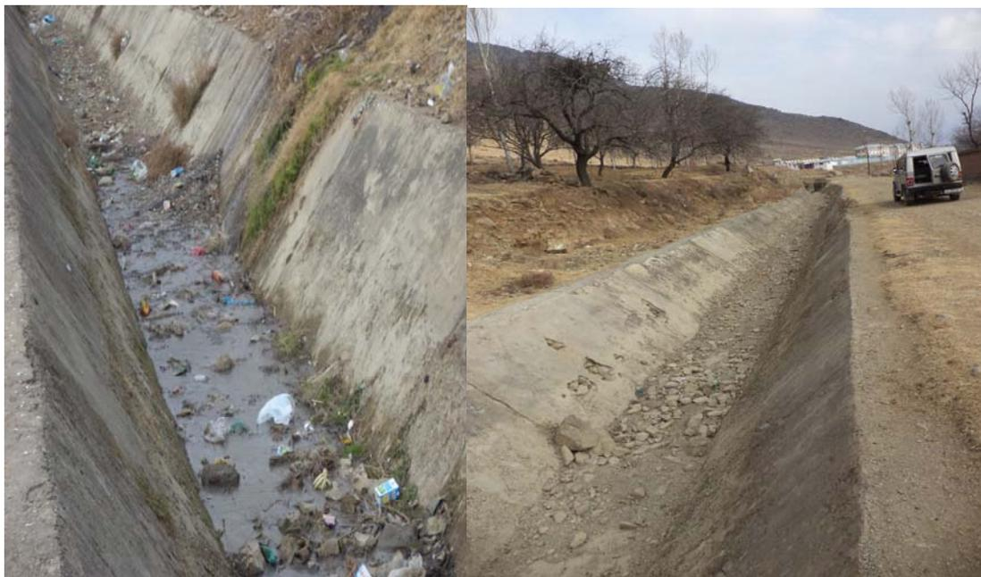
Damages occurred and silt/ garbage accumulated in the Medura canal
