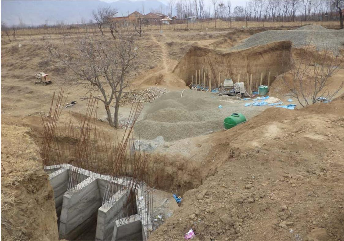
Rajpora canal RCC flume under construction
