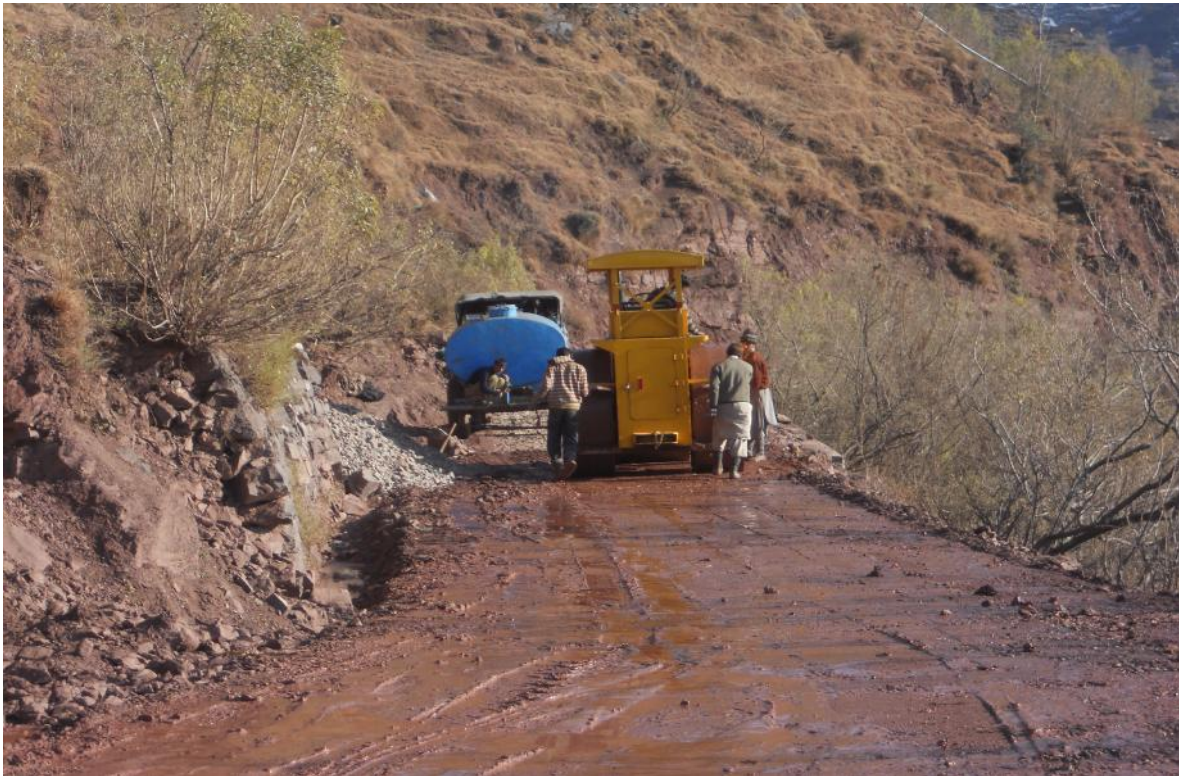
Men & Machinery at work (Mandi side)
