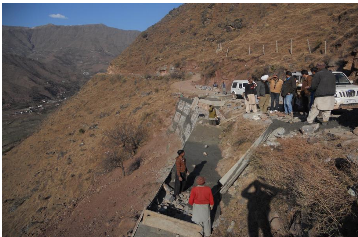
Work on construction of retaining wall under progress
