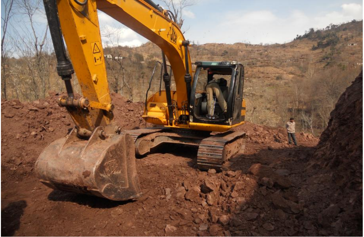
Machinery at work (Buffliaz side)
