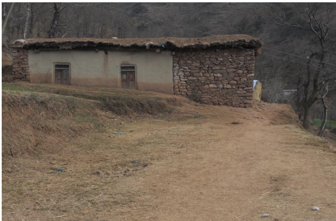
A house structure coming in the alignment of the road
