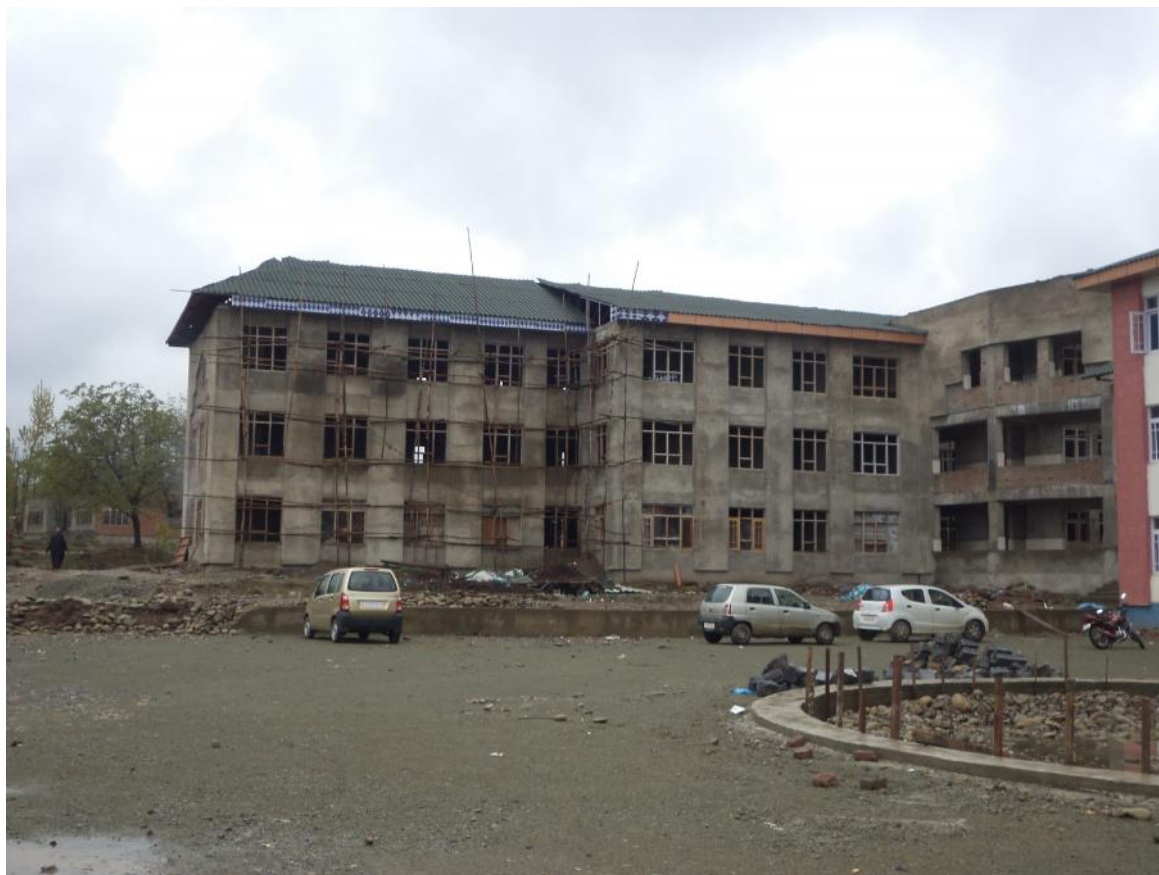
Under construction Western Block
