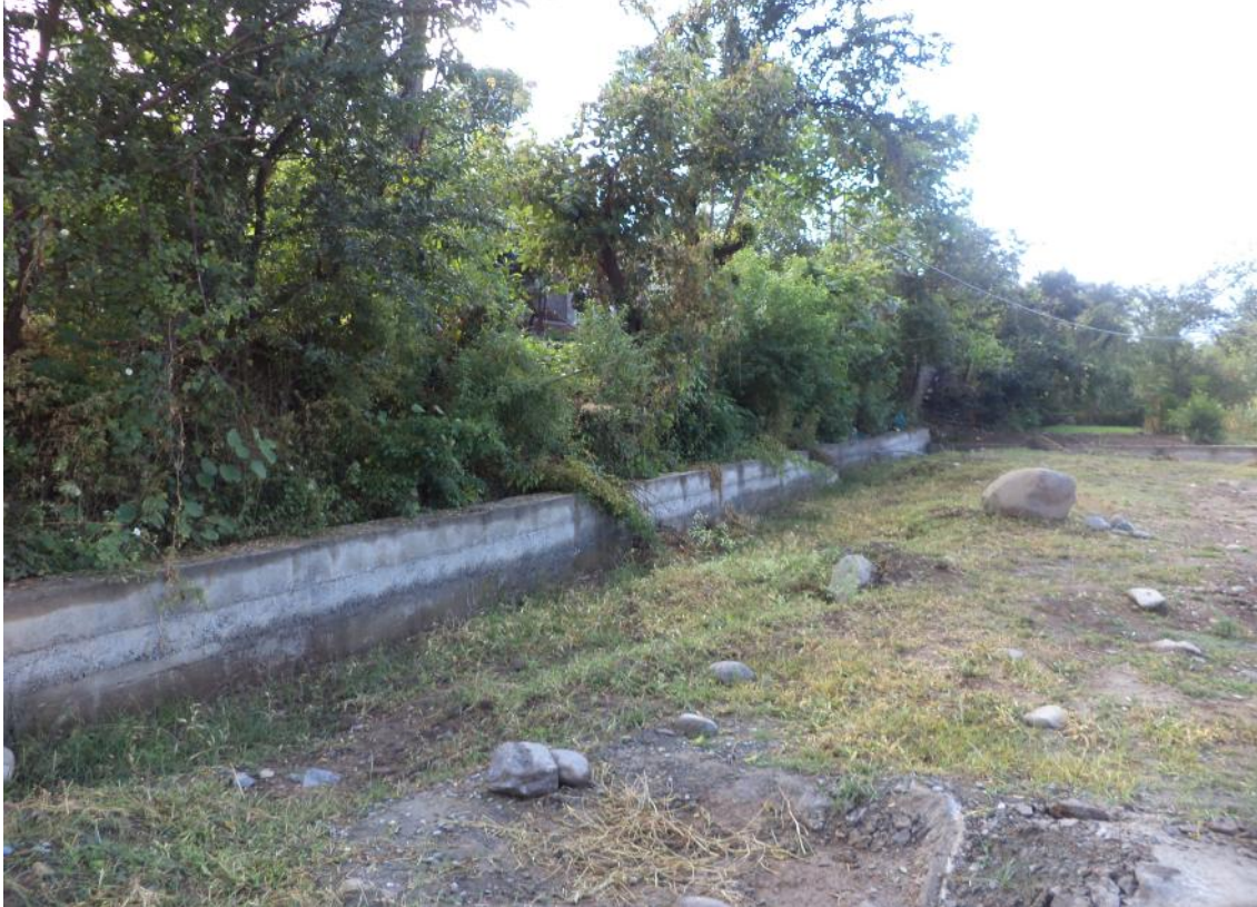
Construction of boundary wall around premises
