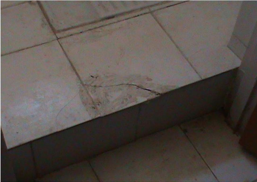
Cracked/broken tiles in the toilet points
