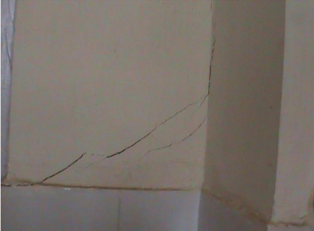
Cracks developed in the walls of the PHC
