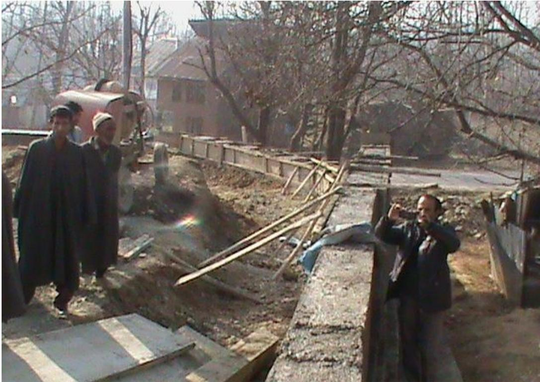
Laying of cement concrete block for boundary wall of PHC under progress
