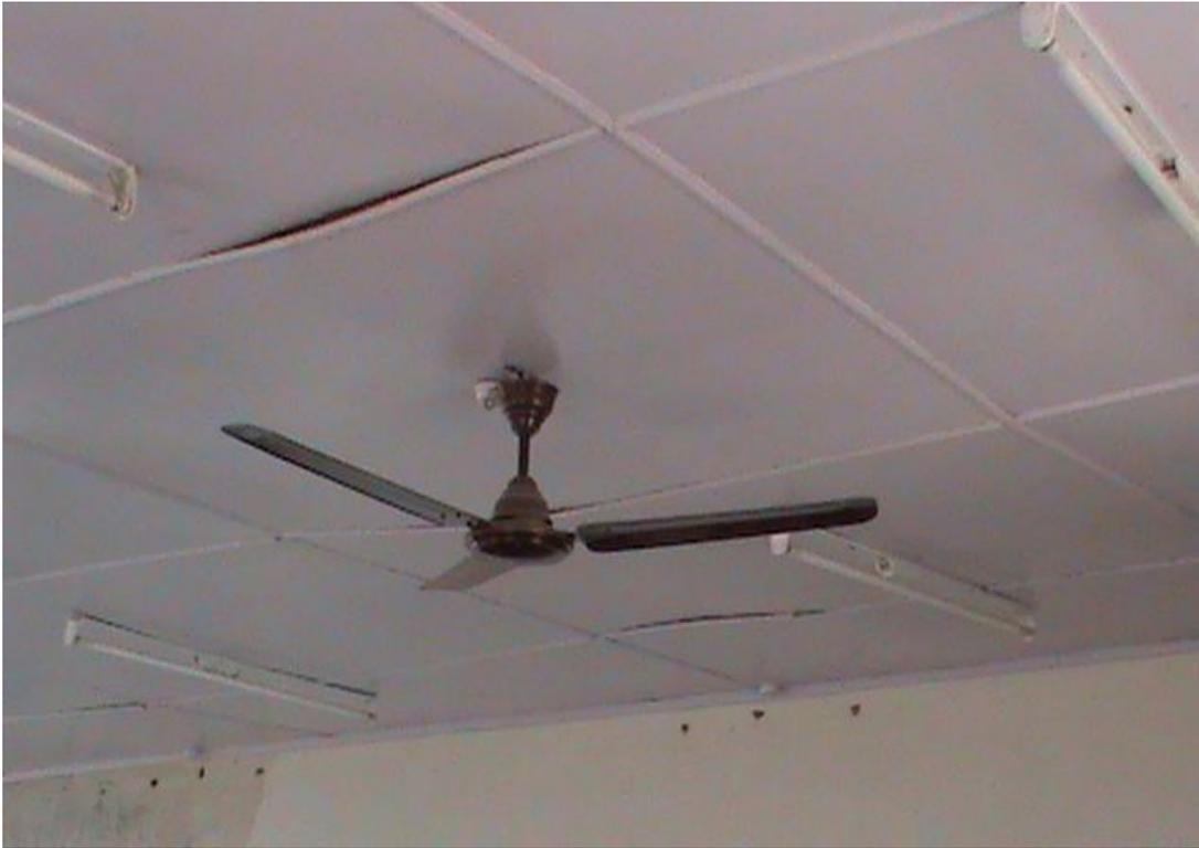
Lack of workmanship quality in fixing of the ceiling
