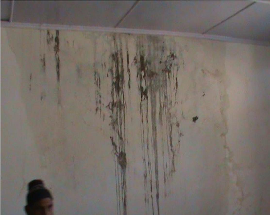
Water leakage/seepage in the walls of PHC
