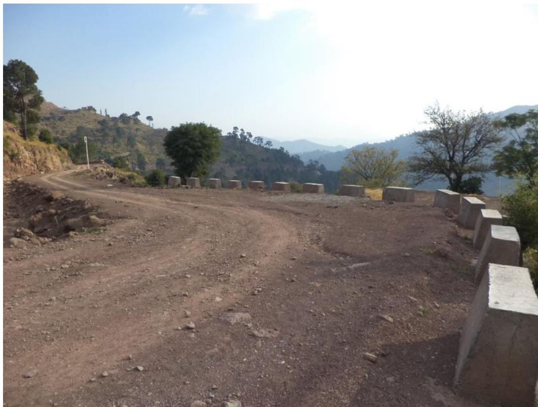
One of the culverts constructed
