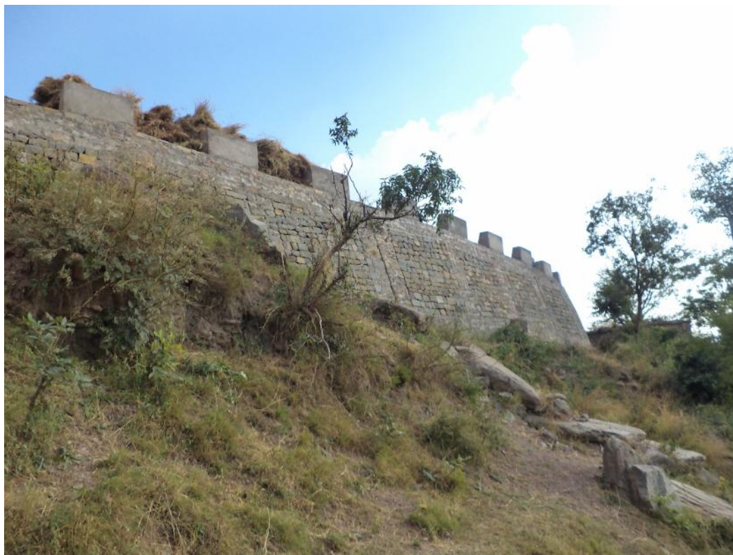
Protection works executed
