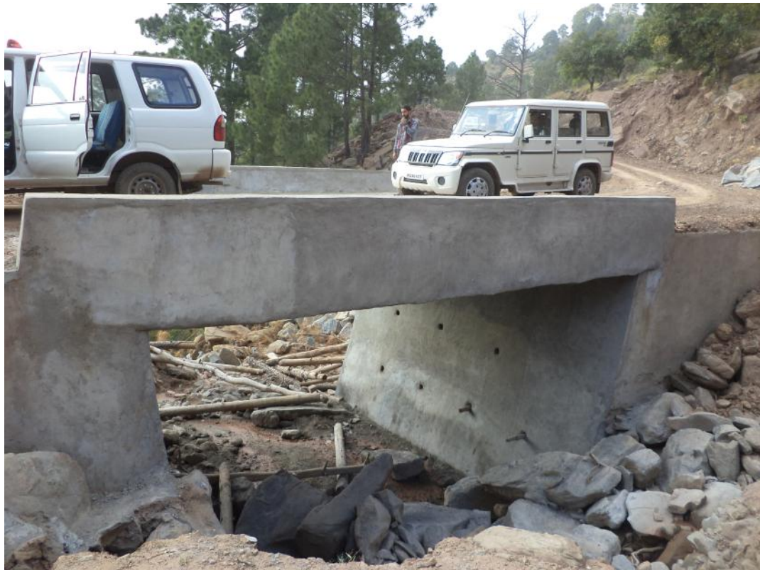
A view of one of the 6 mtr culvert constructed
