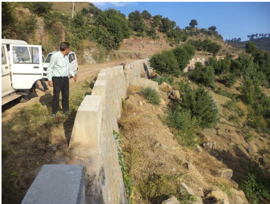
Protection works executed
