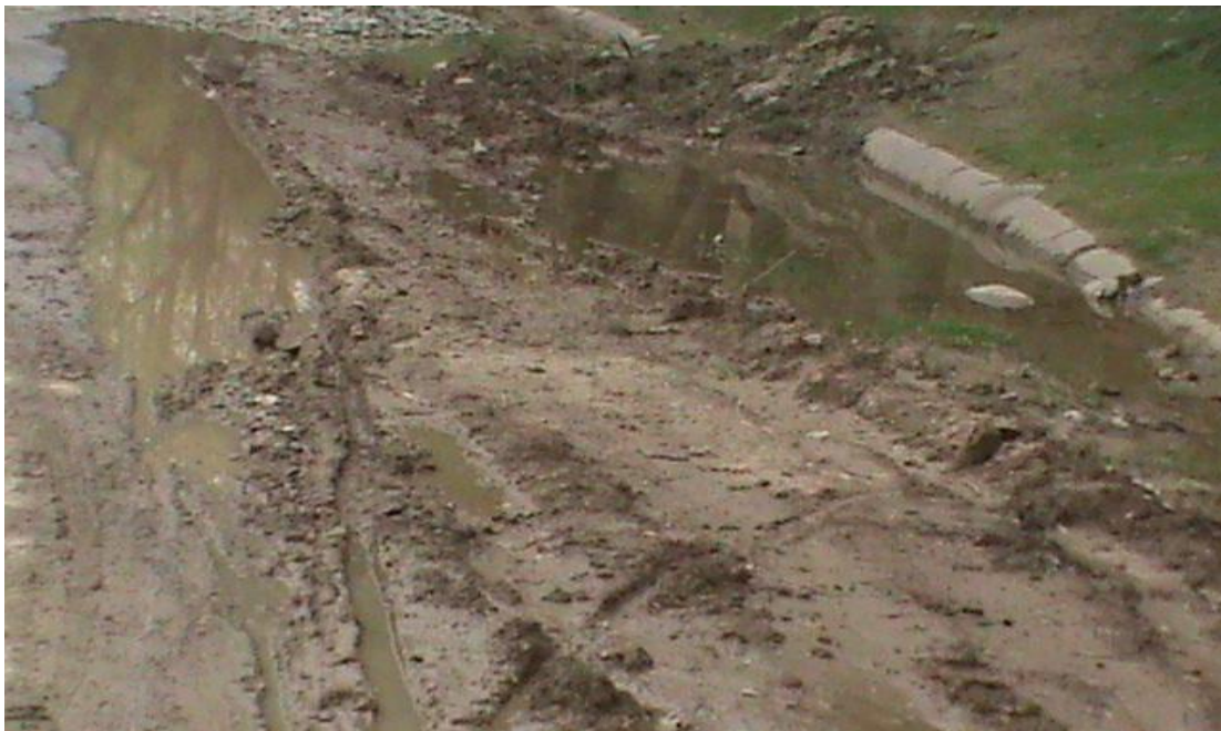
Water supply pipes leaking at the joints
