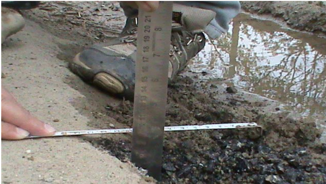
Checking thickness of the BM and OGP
