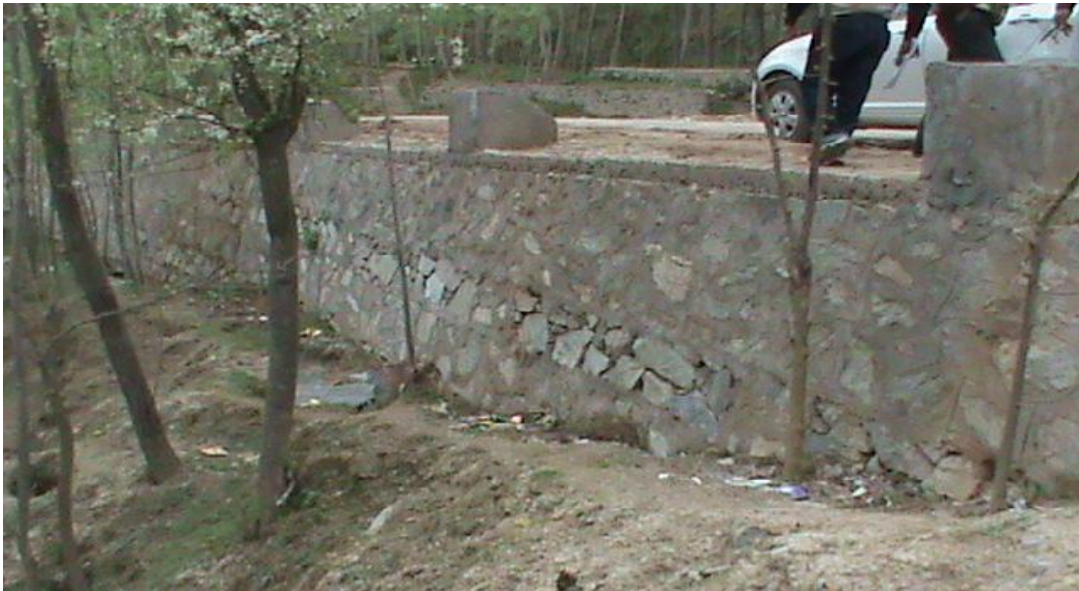
Retaining wall constructed near on Km 2 nd of the road
