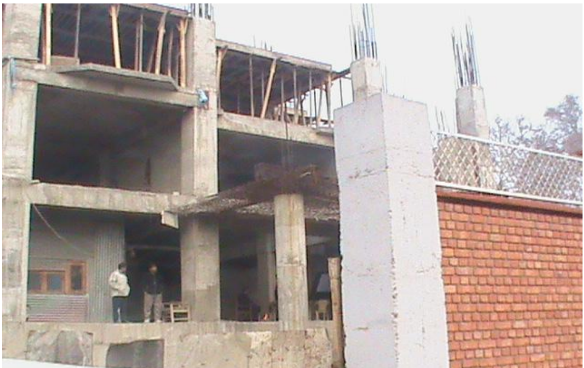
Shuttering on 3 rd floor slab in progress
