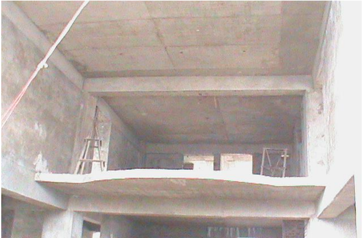
Inner view of cement plastered mezzanine floors
