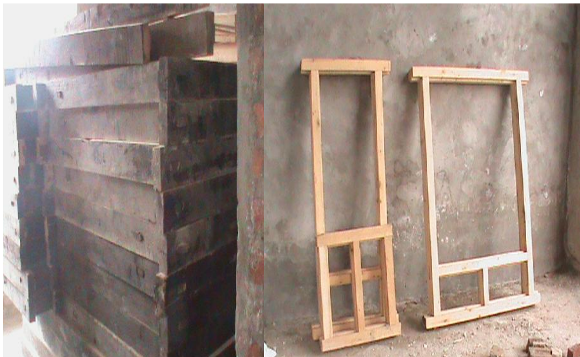
Window/Door frames made of Deodar, ready for fixing
