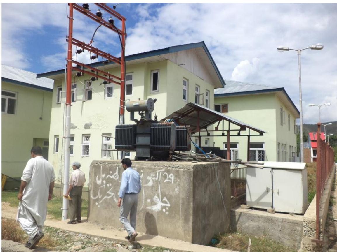
630 KVA Electric Sub-Station created within the SDH premises
