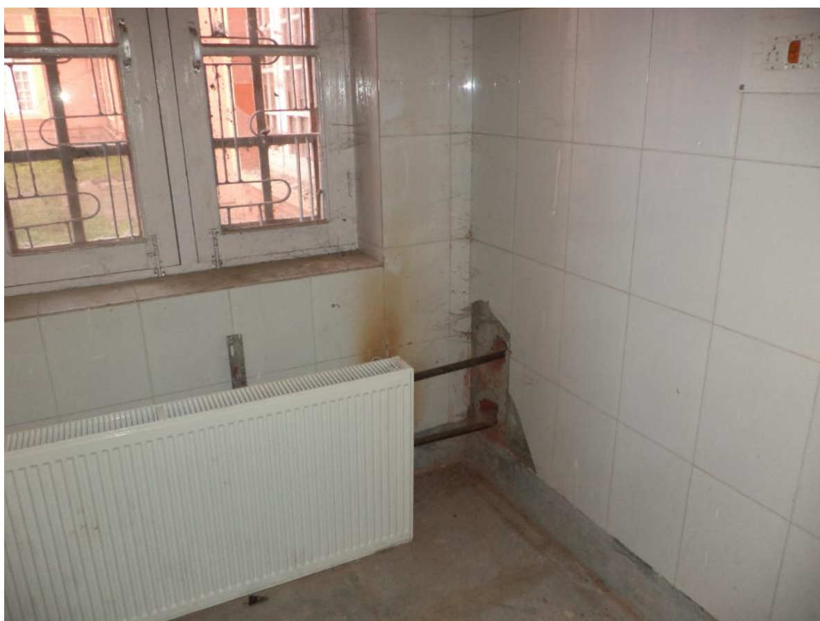
Damage to the walls due to Central Heating System work
