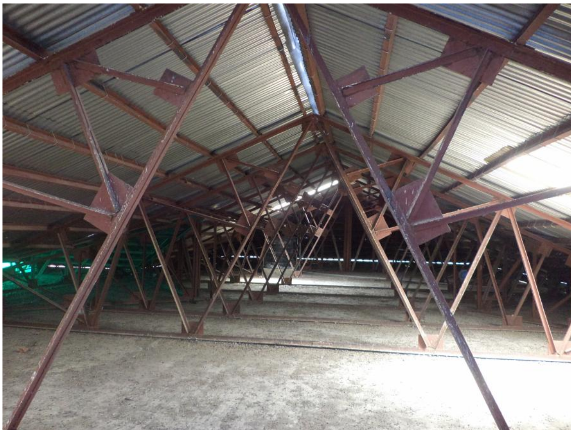
Steel truss work of the main hospital building
