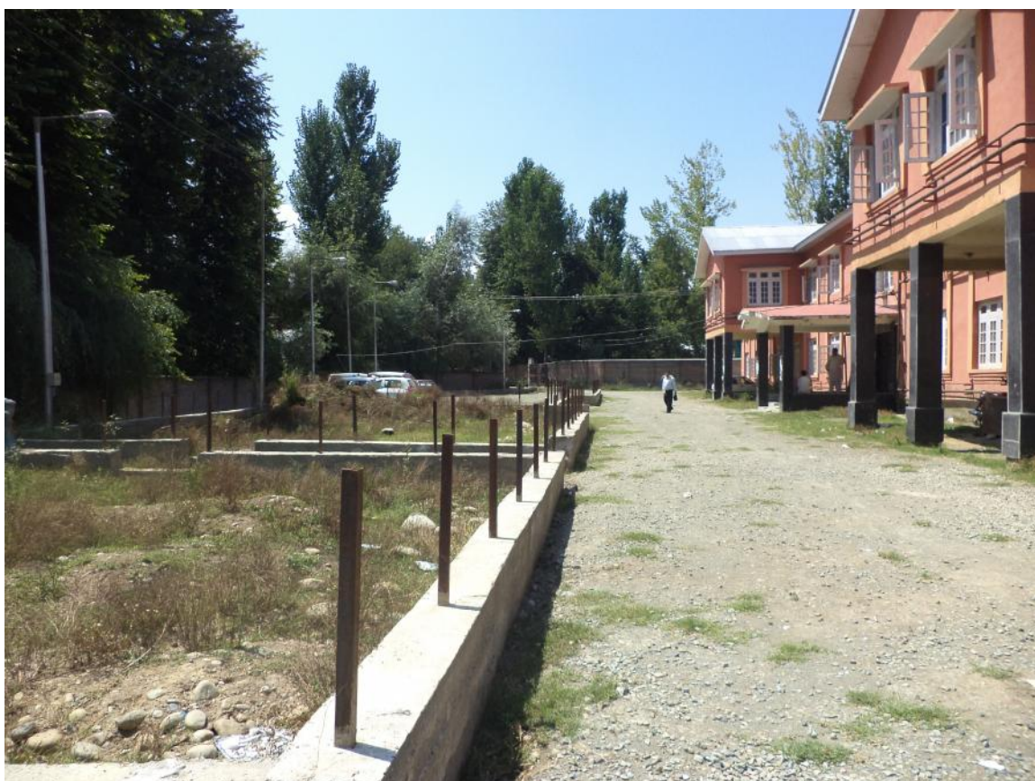
Site development works under progress
