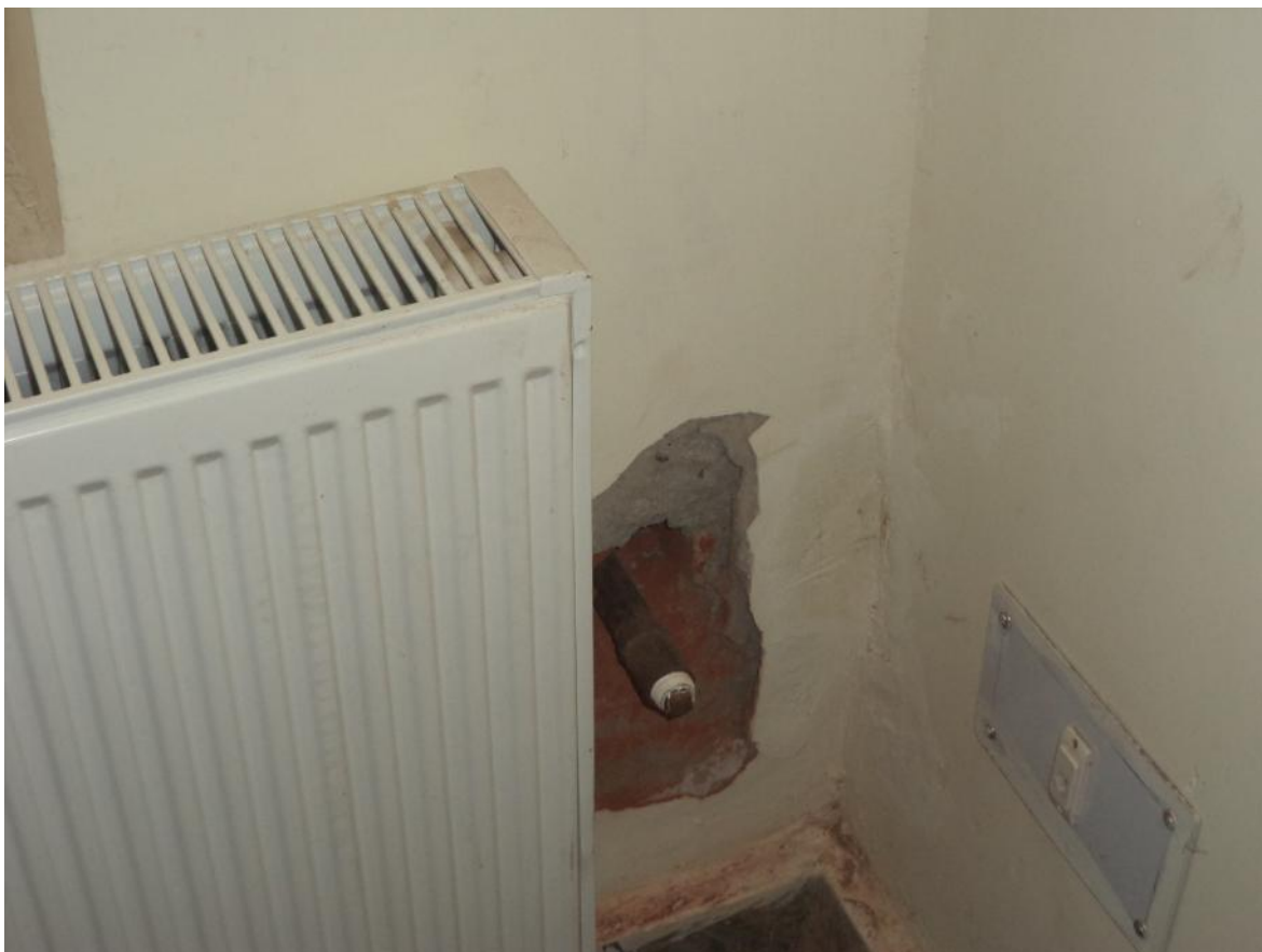
Damage to the walls due to Central Heating System work
