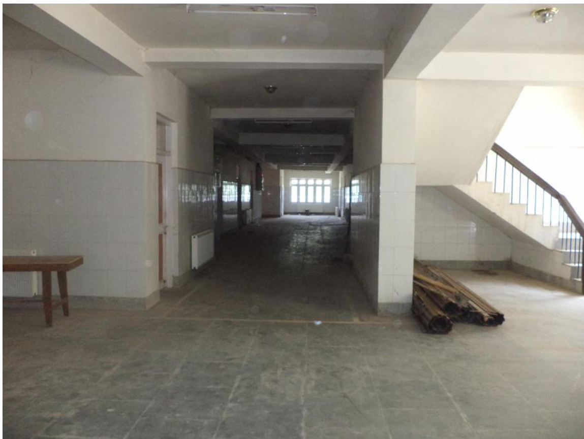
View of the hospital corridor in the ground floor
