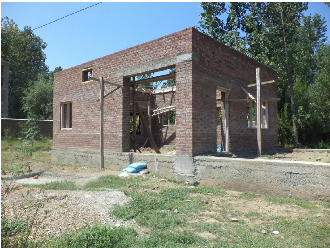
Boiler House for Central Heating System under construction
