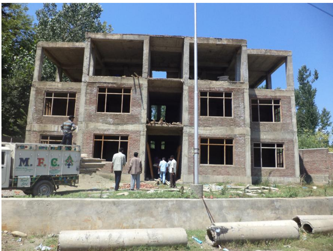
Doctors' quarter under construction
