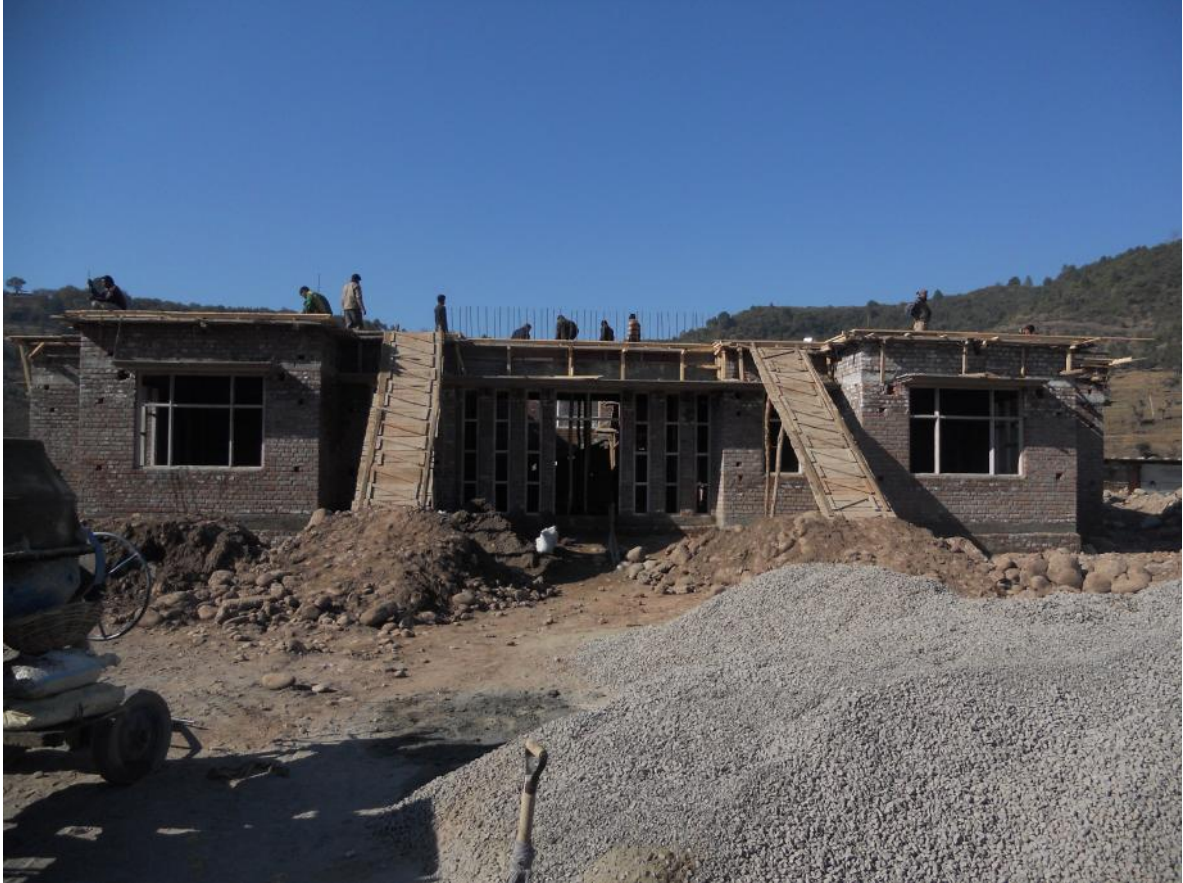
Administrative Block—under construction at TFC
