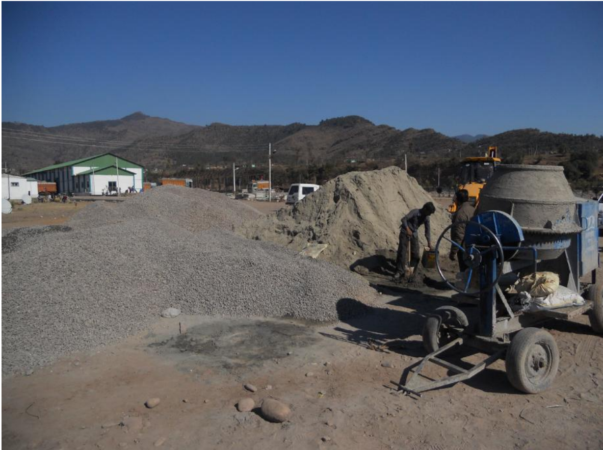
Men & Machinery working at the project
