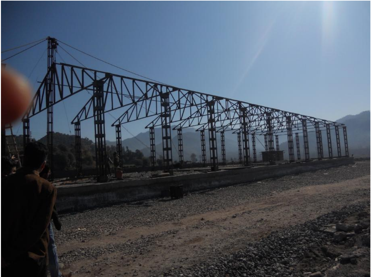
Open Cargo Platform under Construction
