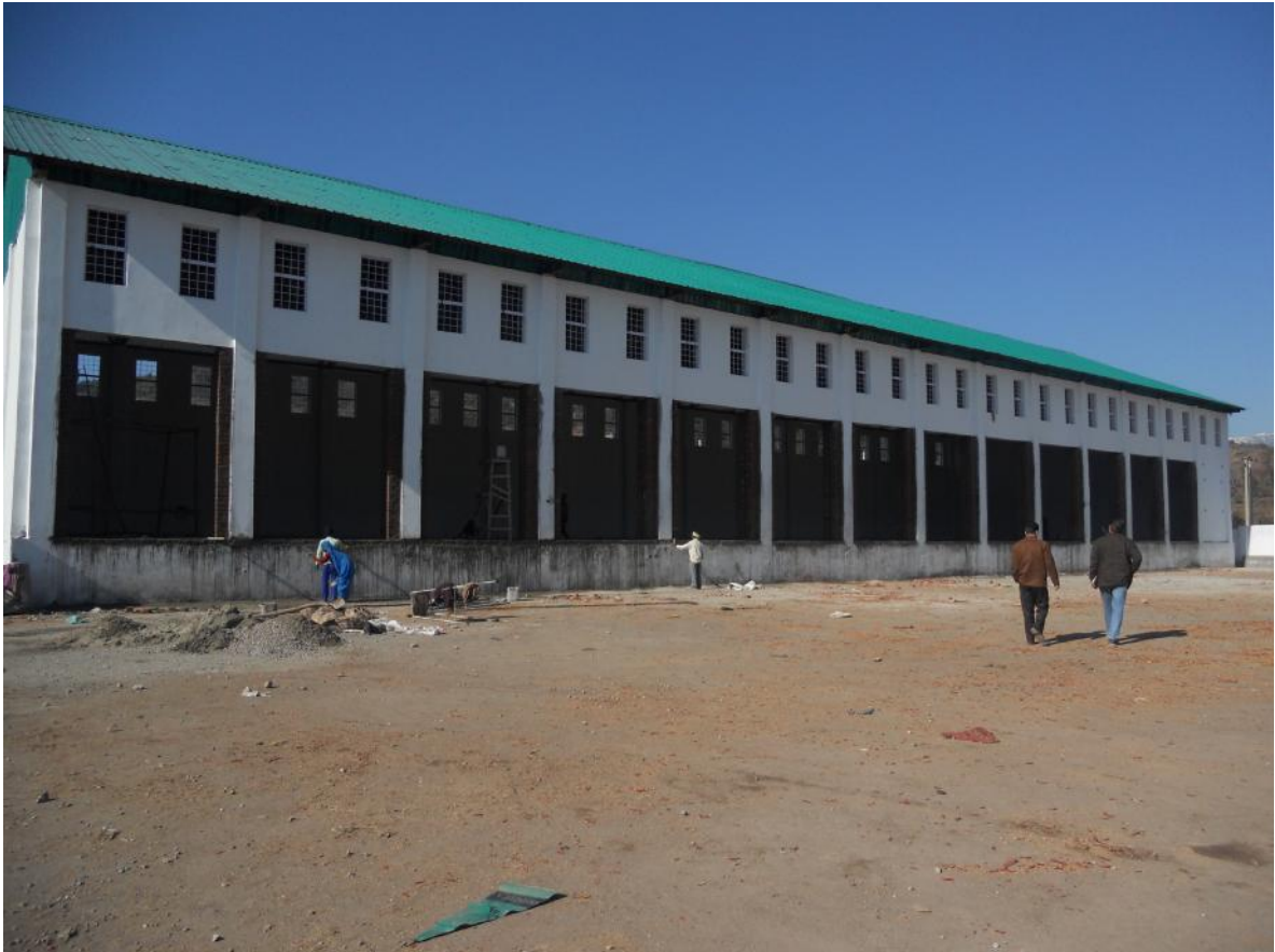
Newly constructed Godown with 13 Shutters
