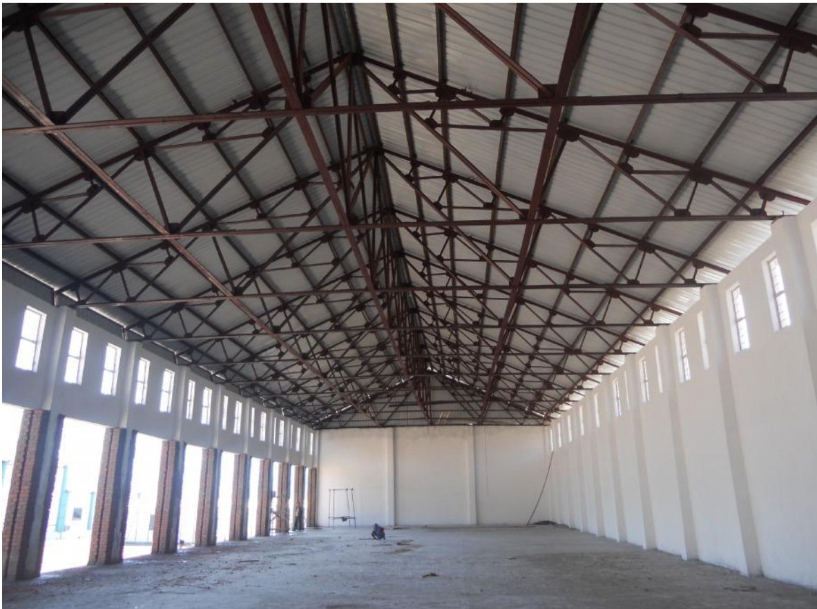
Inner view of the newly constructed Godown
