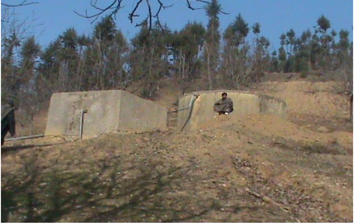
Service Reservoir of the old Water Supply Scheme at Batpora
