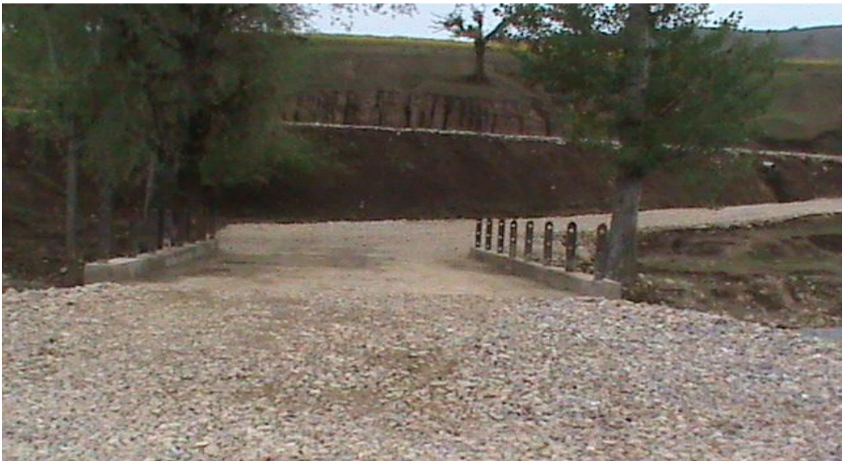
Approach road (near Parthan) to site of Treatment Plant
