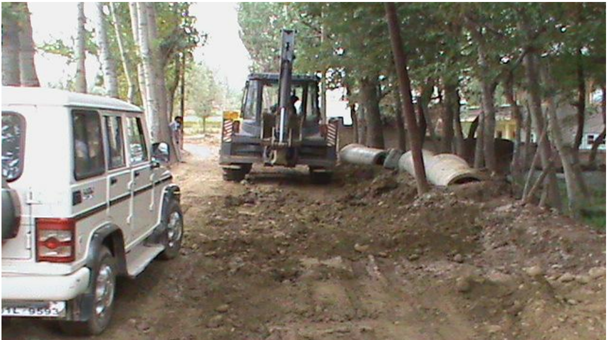
Road restoration work in progress at Watrewani
