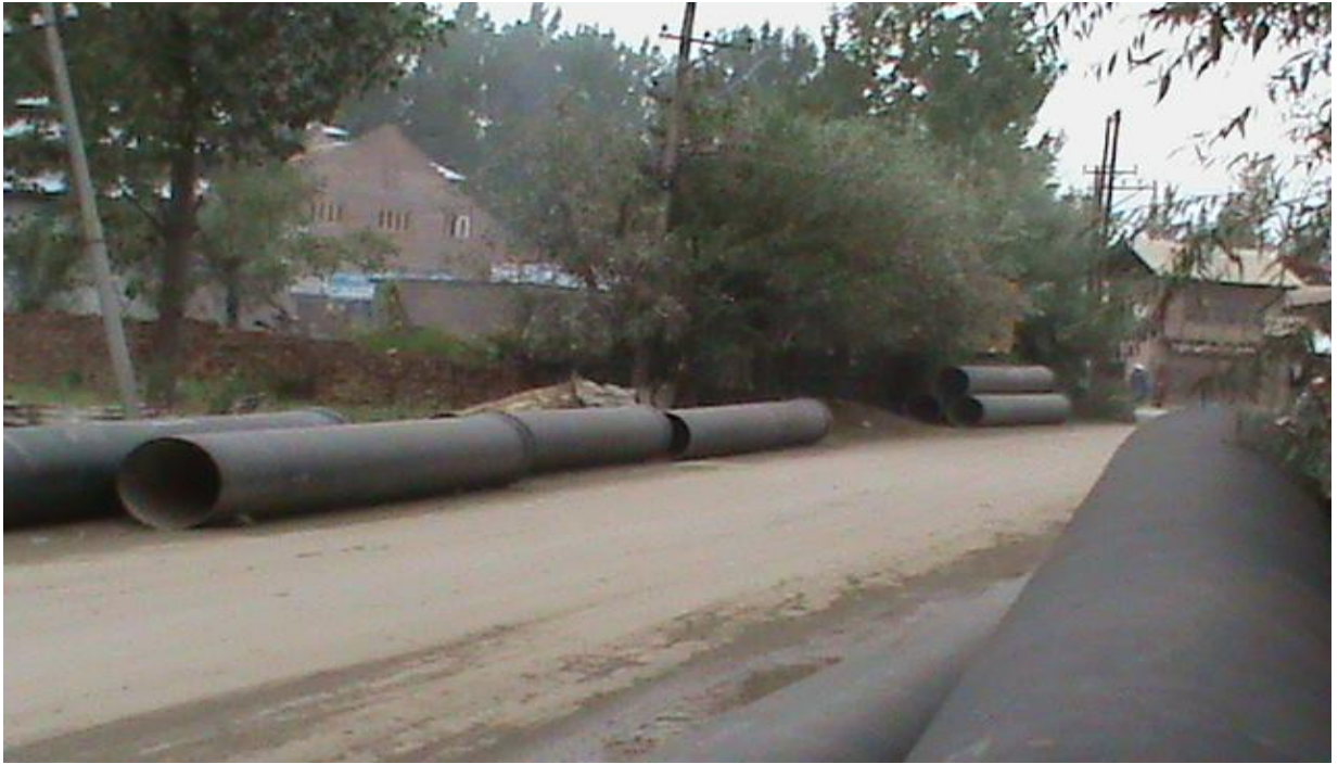
Pipes dumped along the road side
