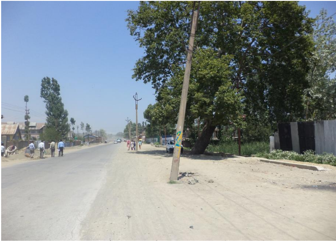
Non-usable electric poles still existing on road
