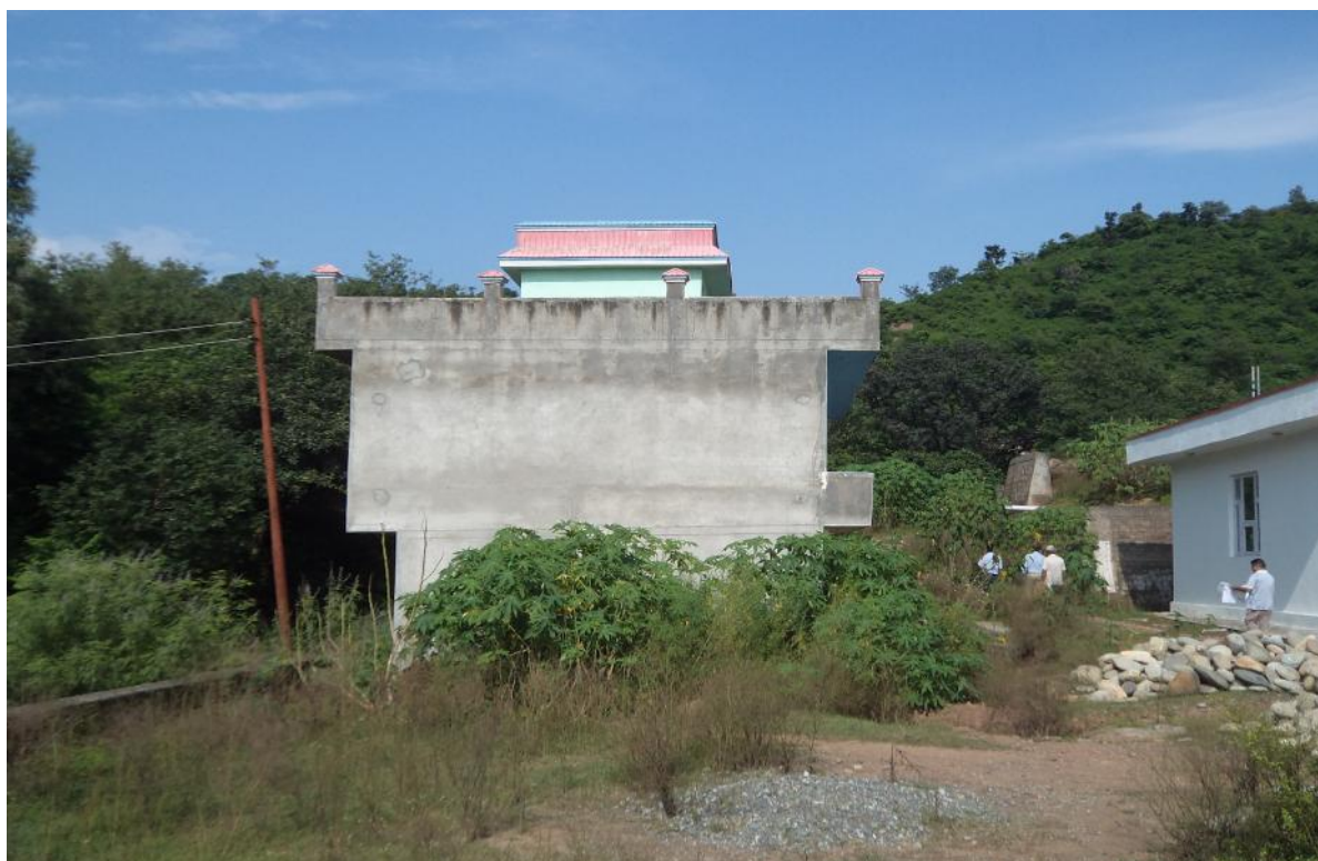
Side View indicates the buildings intrusion into the CHC Complex
