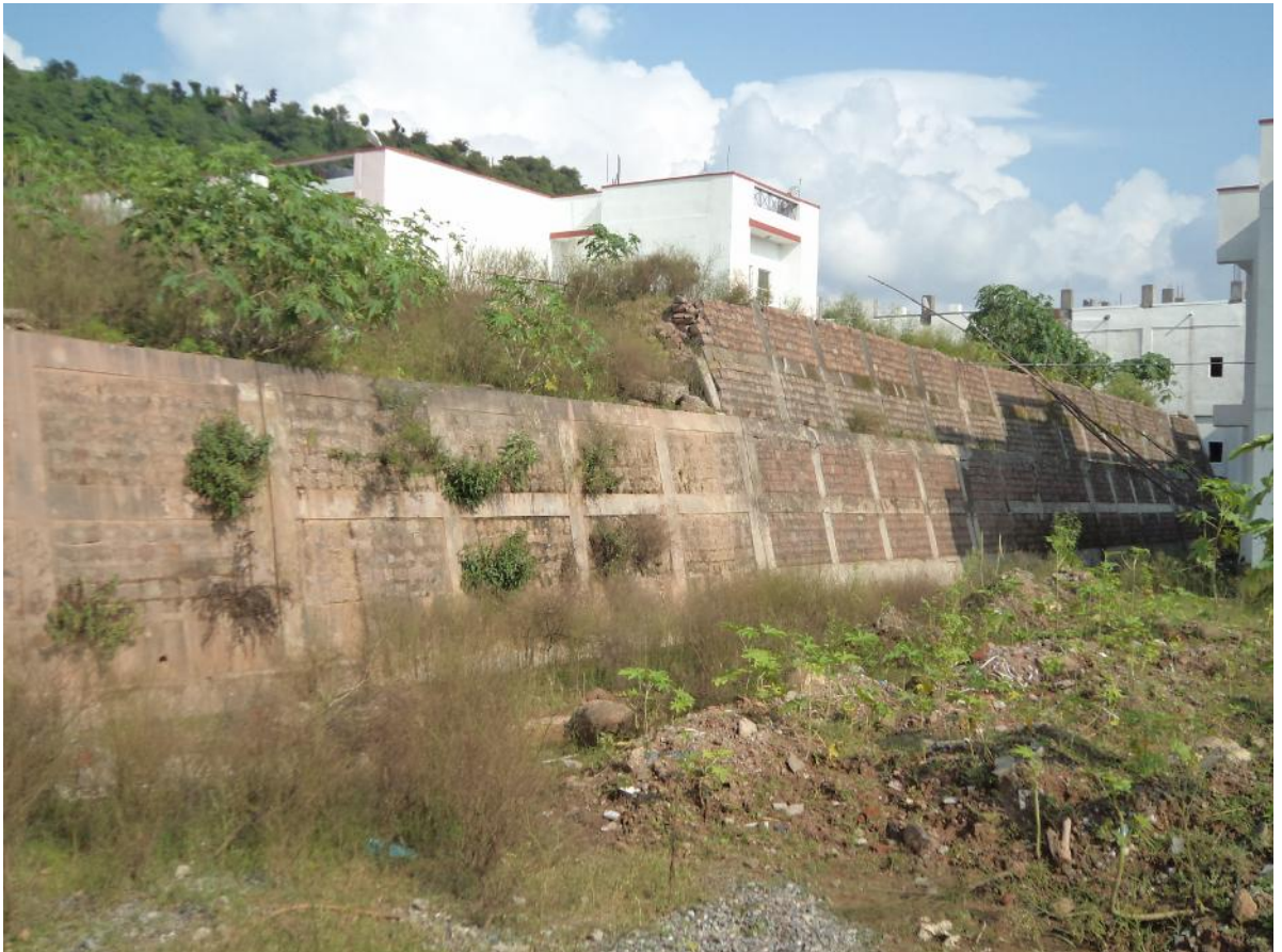
Retaining Wall between the IPD and OPD Blocks
