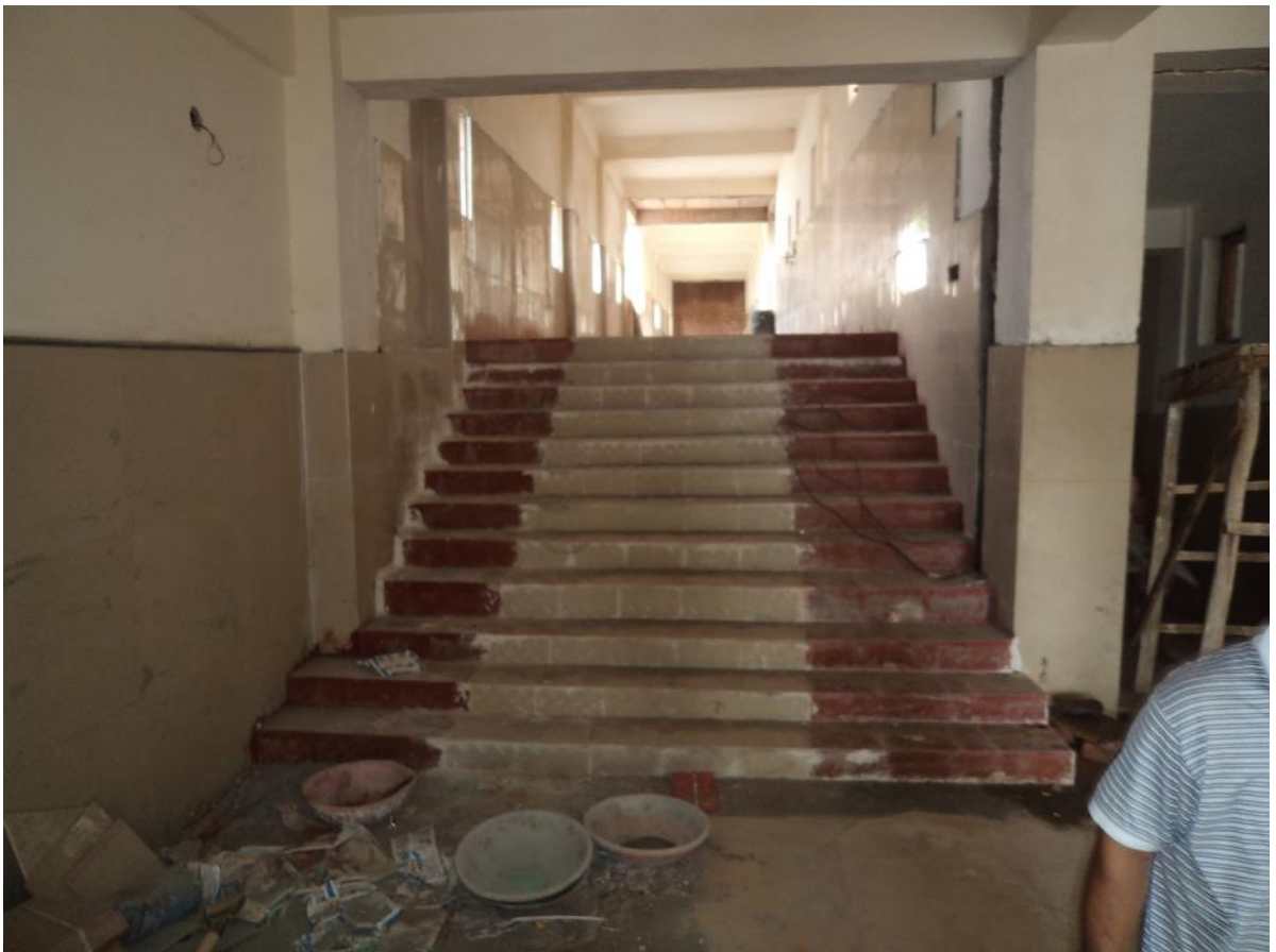
Connecting Corridor between IPD and OPD Block
