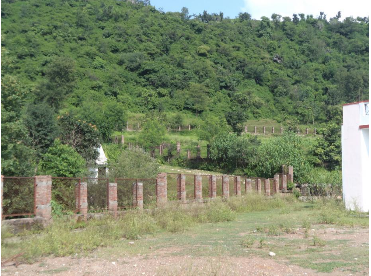
Boundary Fencing of CHC complex
