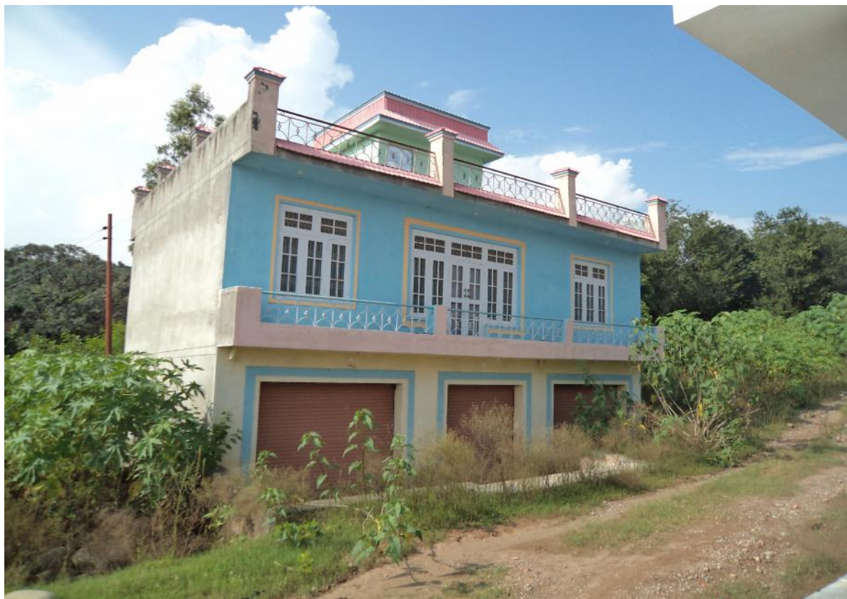
Structure Constructed by Ex MLA along CHC Boundary Fence
