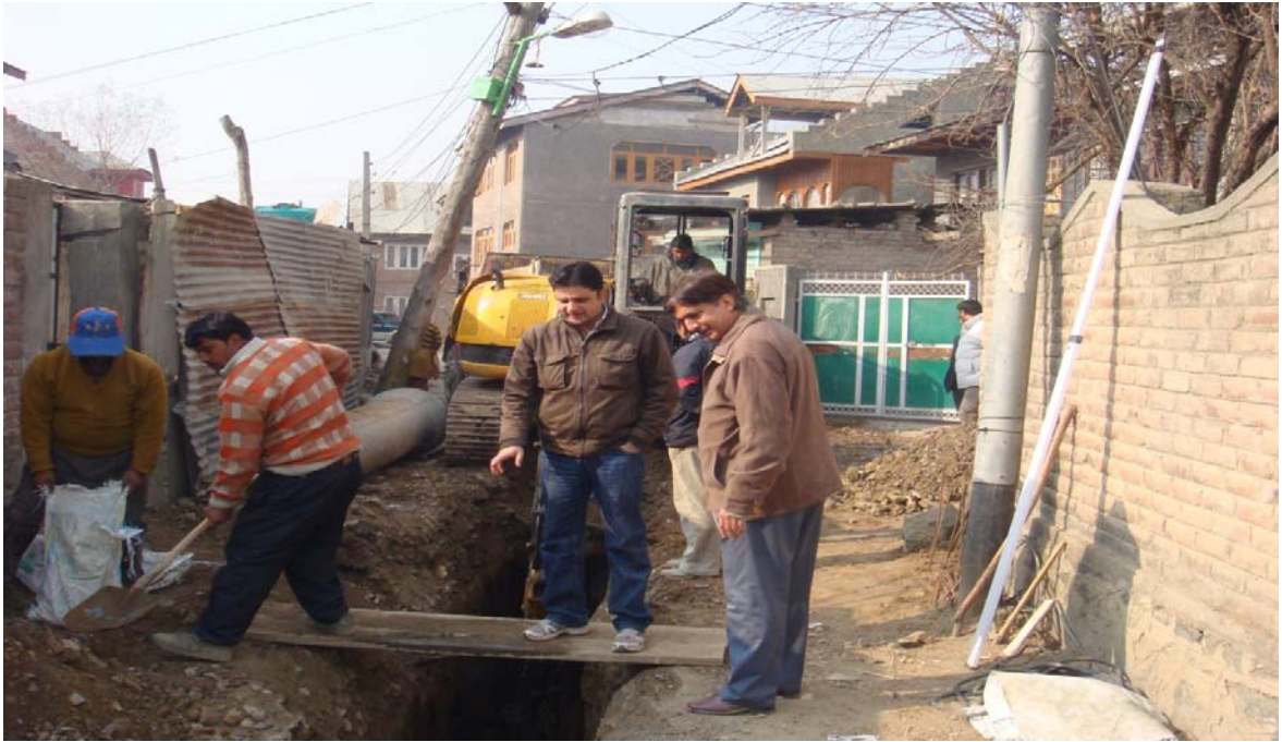
Laying of lateral sewer pipe line at Zoonimar Ali Jan road
