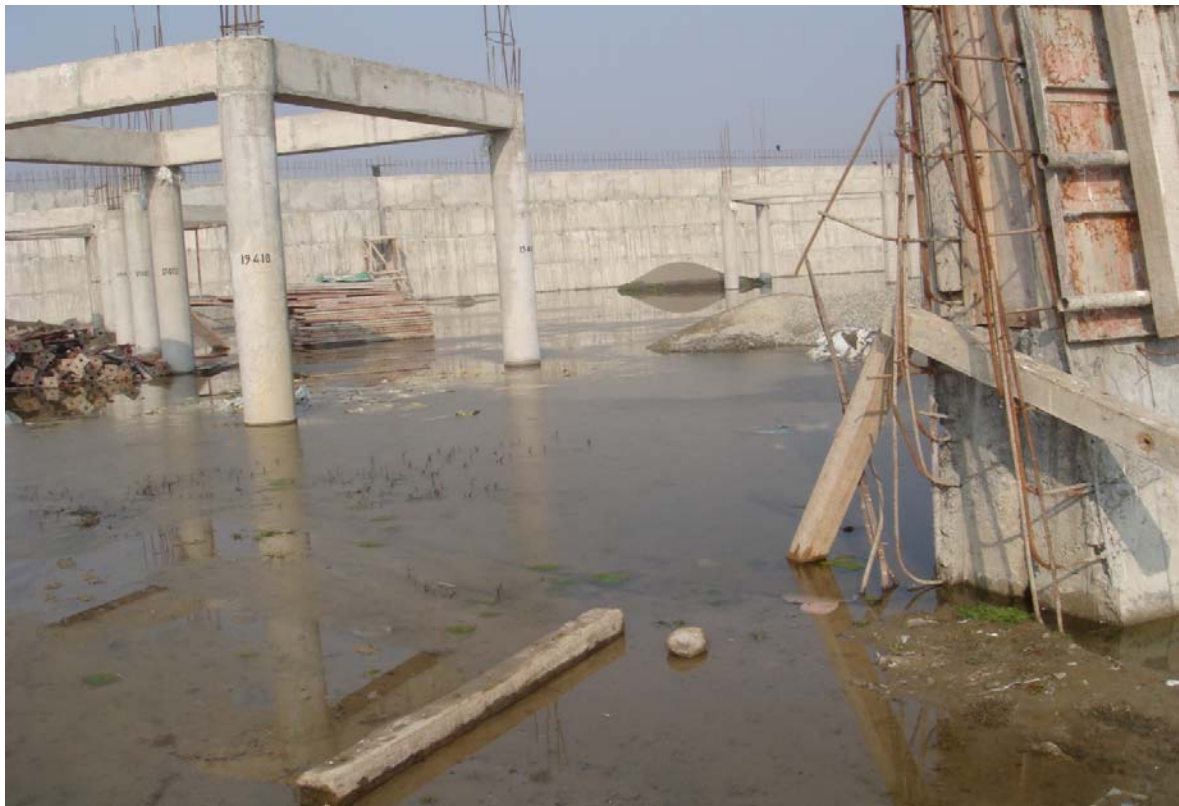
Construction site of STP at Noorbagh, Srinagar
