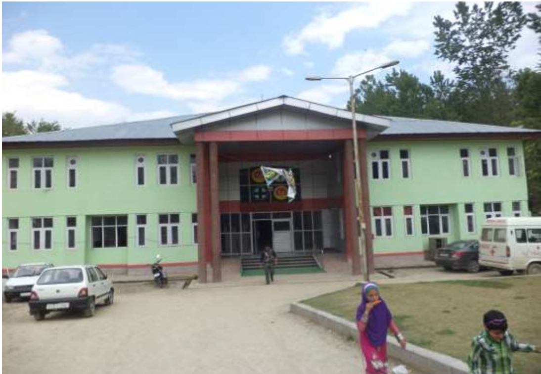
Front view of the SDH building
