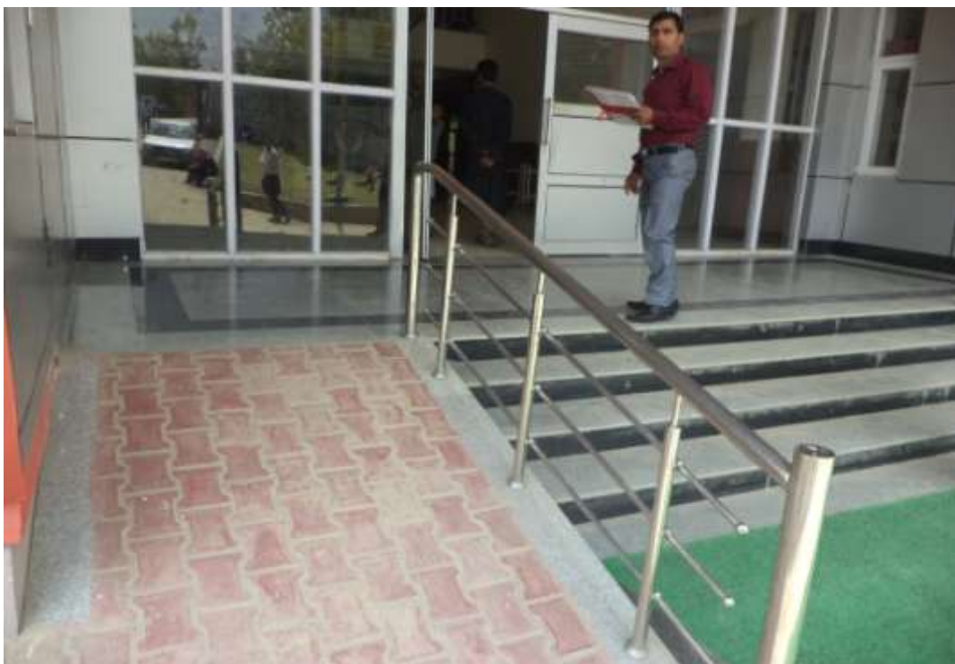
Stainless steel railings fixed along ramp on the entrance
