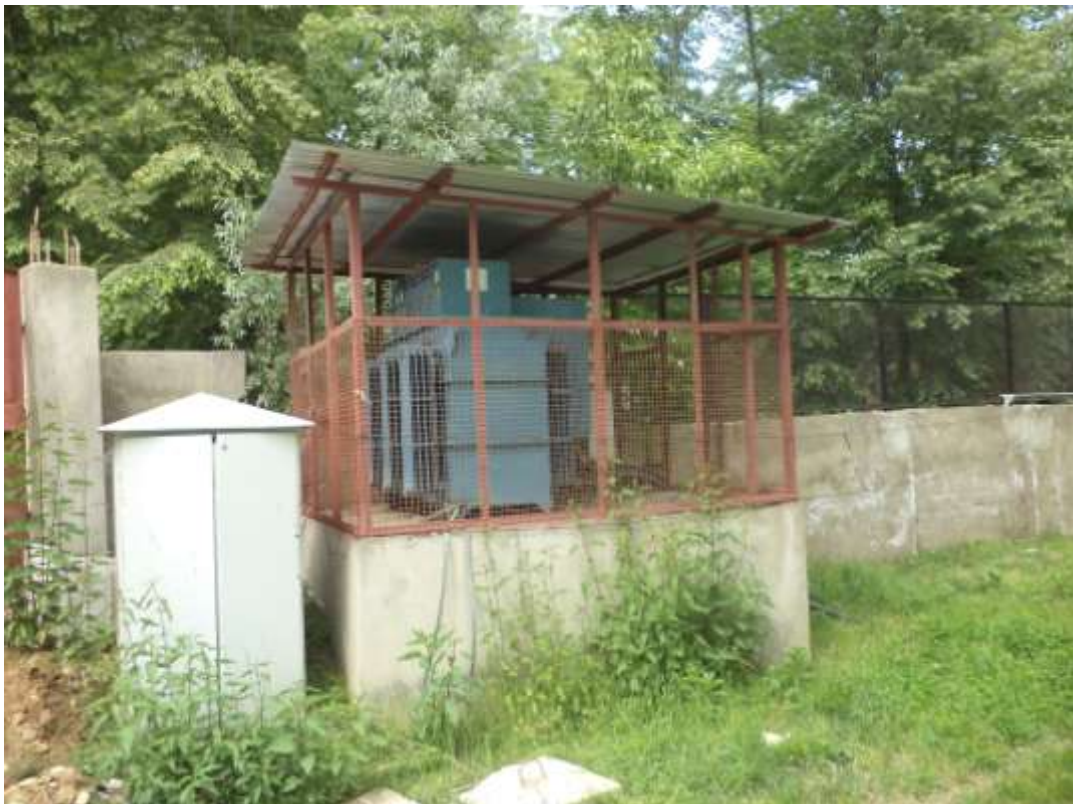
Installation of AVR (400 KVA capacity) within the premises of hospital
